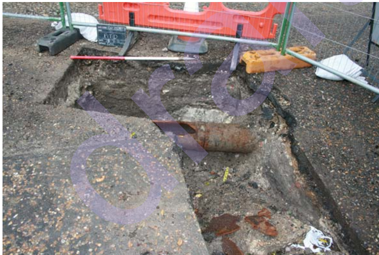
Plate 4. Trench D facing west
