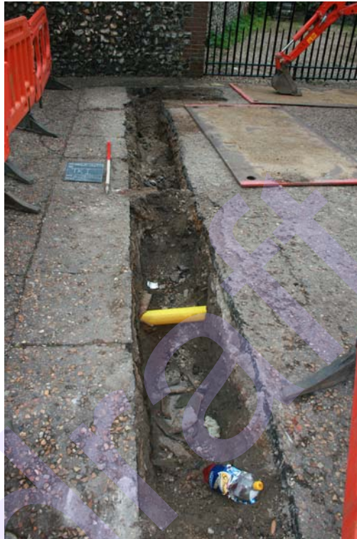
Plate 9. Trench I facing south
