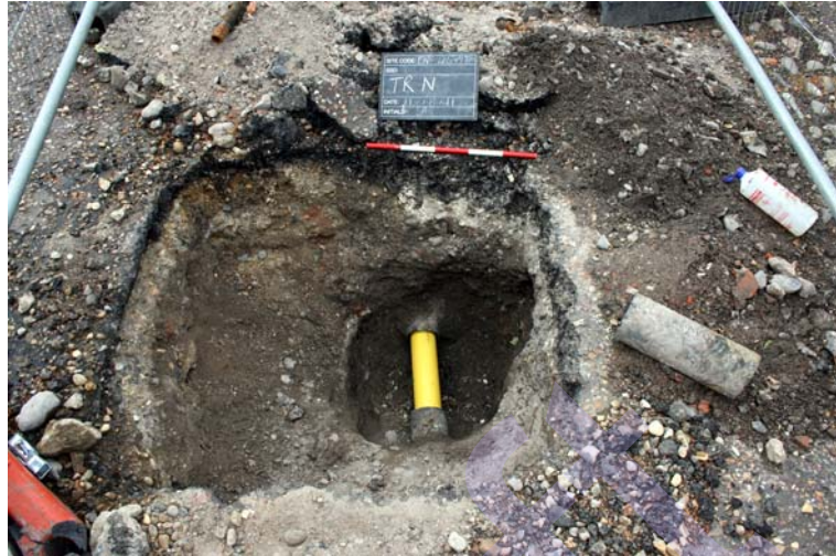
Plate 14. Trench N facing west
