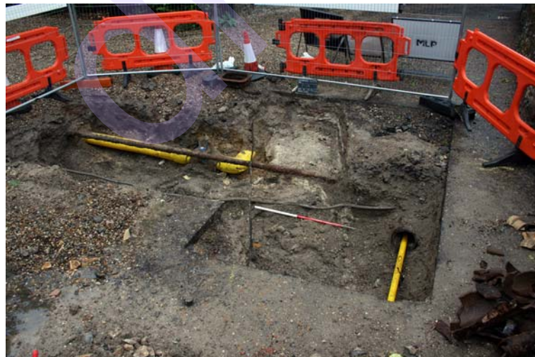
Plate 1. Trench A facing north
