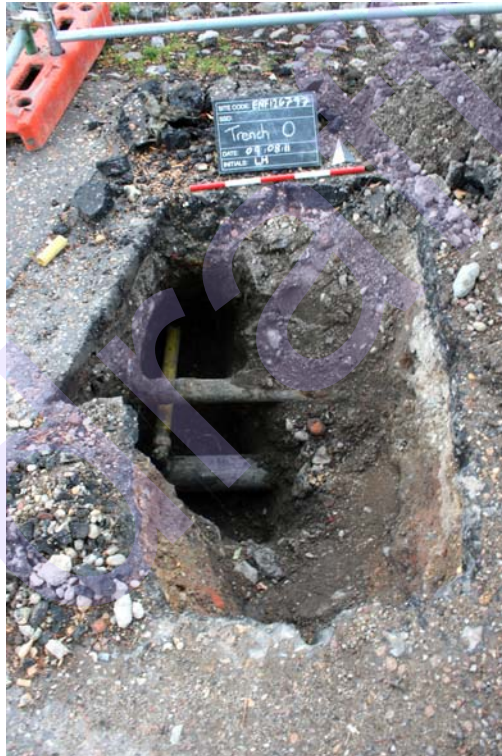
Plate 15. Trench O facing north
