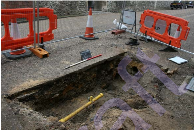
Plate 3: Trench C facing northwest
