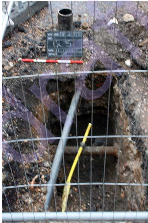
Plate 19. Trench S facing south
