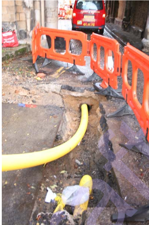
Plate 34. Trench SS facing west
