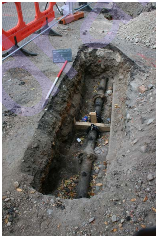
Plate 11. Trench K facing west
