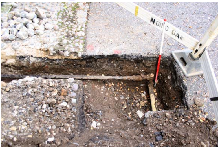
Plate 35. Trench TT facing north
