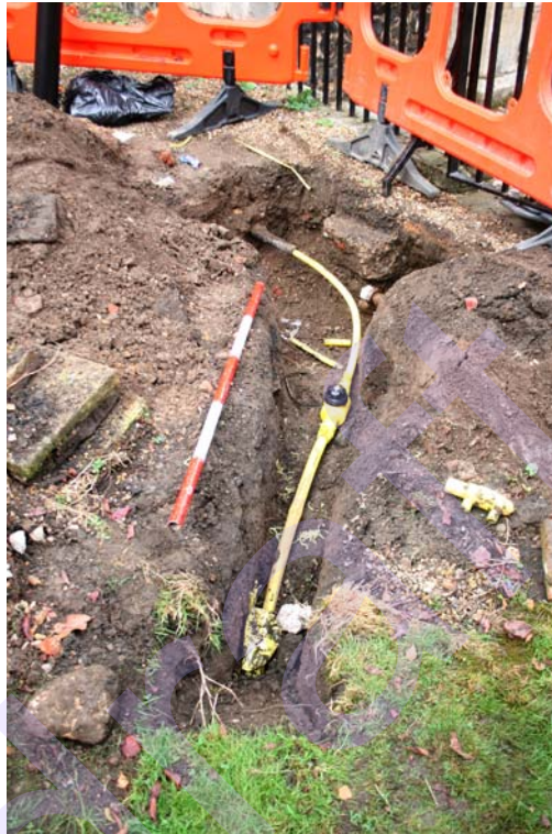
Plate 30. Trench GG facing north-west
