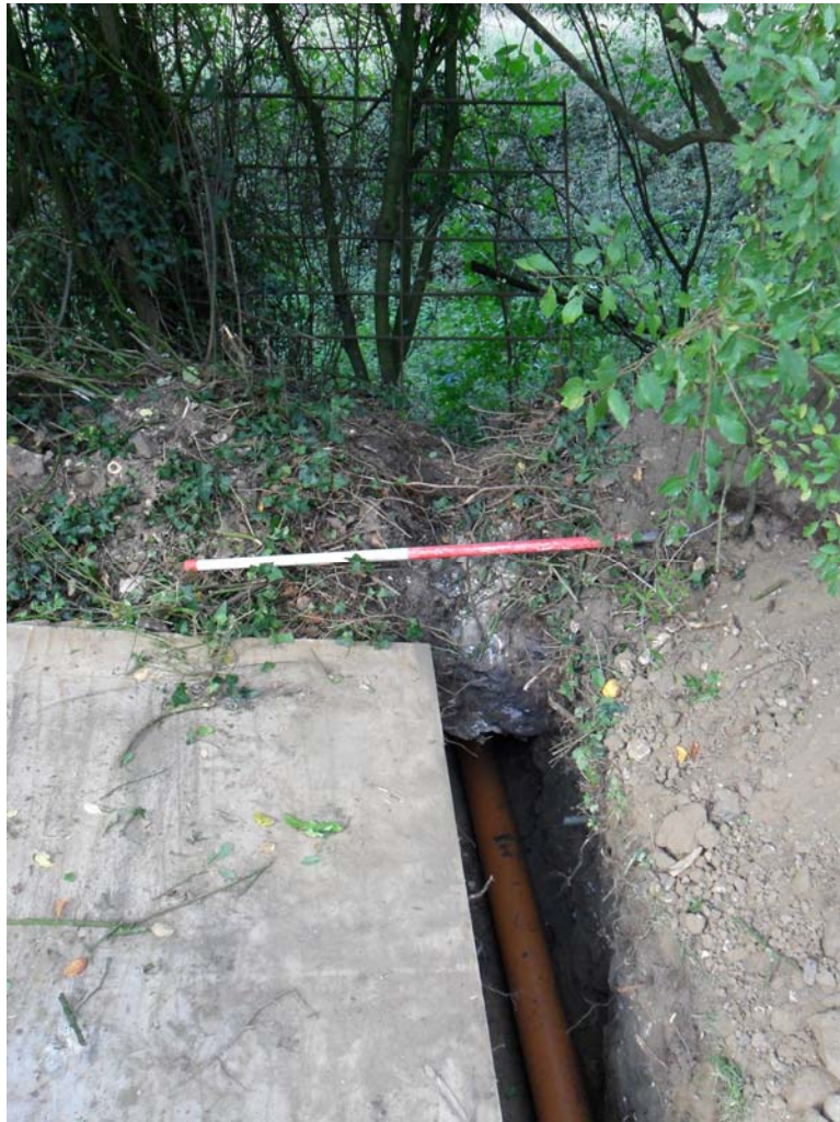
Plate 9. The trench through the bank and into the 'hollow way'
