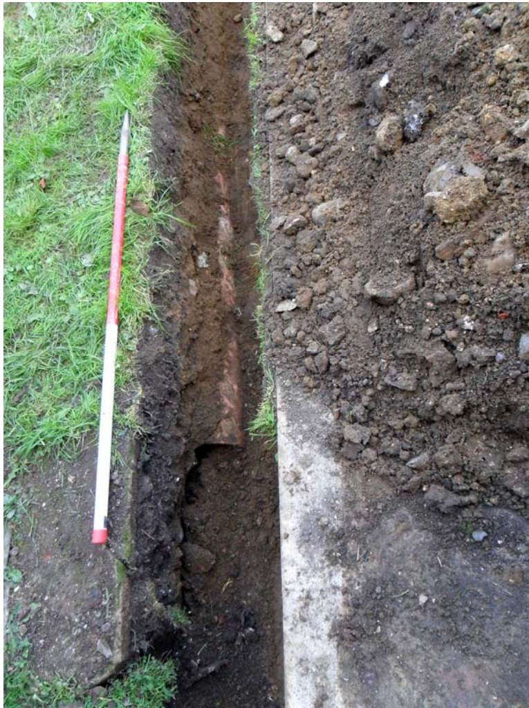
Plate 1. Trench from downpipe into Inspection Pit 1
