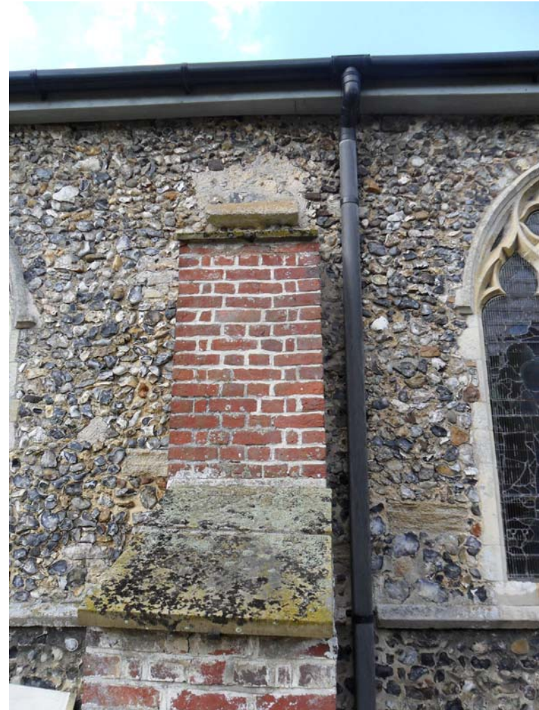
Plate 5. Red brick replacement buttress, showing location of original
