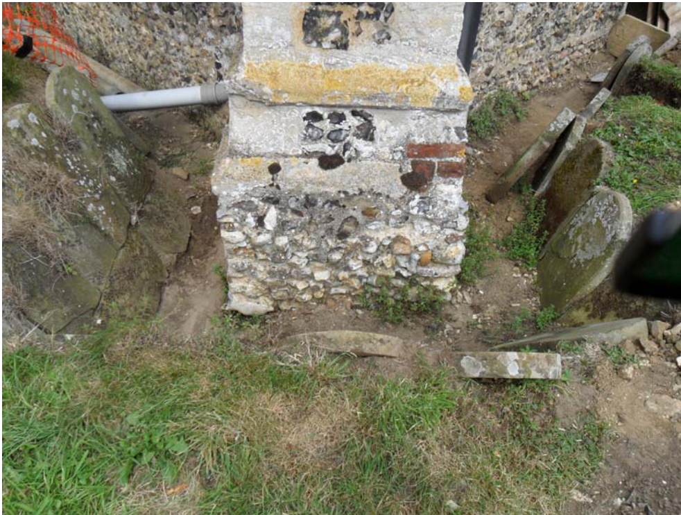
Plate 8. Headstone arrangement around former drainage works
