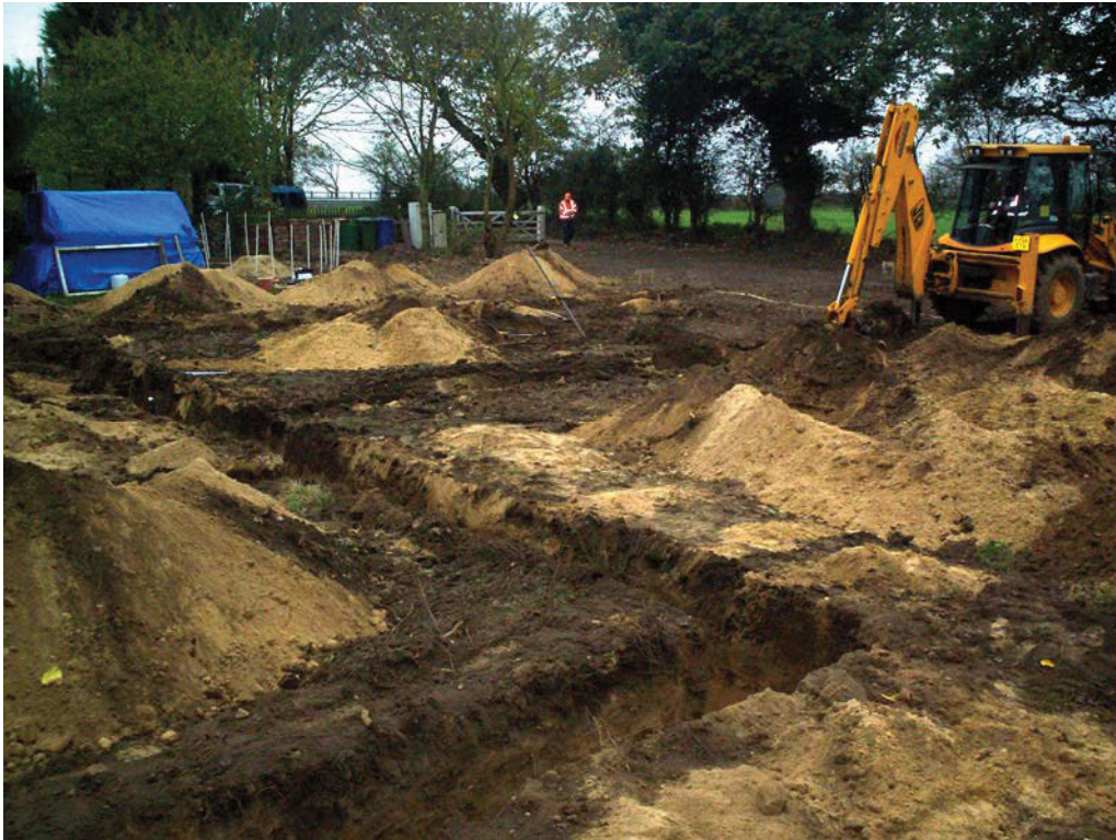
Plate 1. Foundations facing north-west
