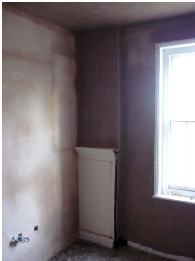
Plate 2. Bedroom 2 showing the repositioned wall splitting the chimney breast and fireplace.
