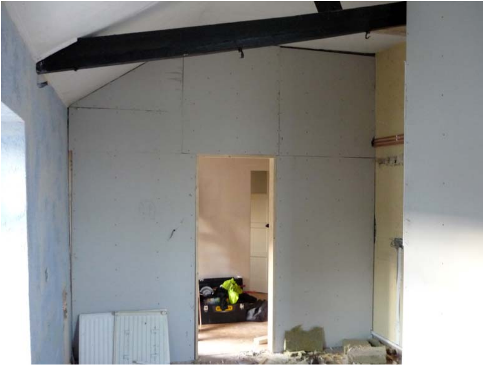
Plate 1. The new stud and plasterboard north-east wall in the kitchen.
