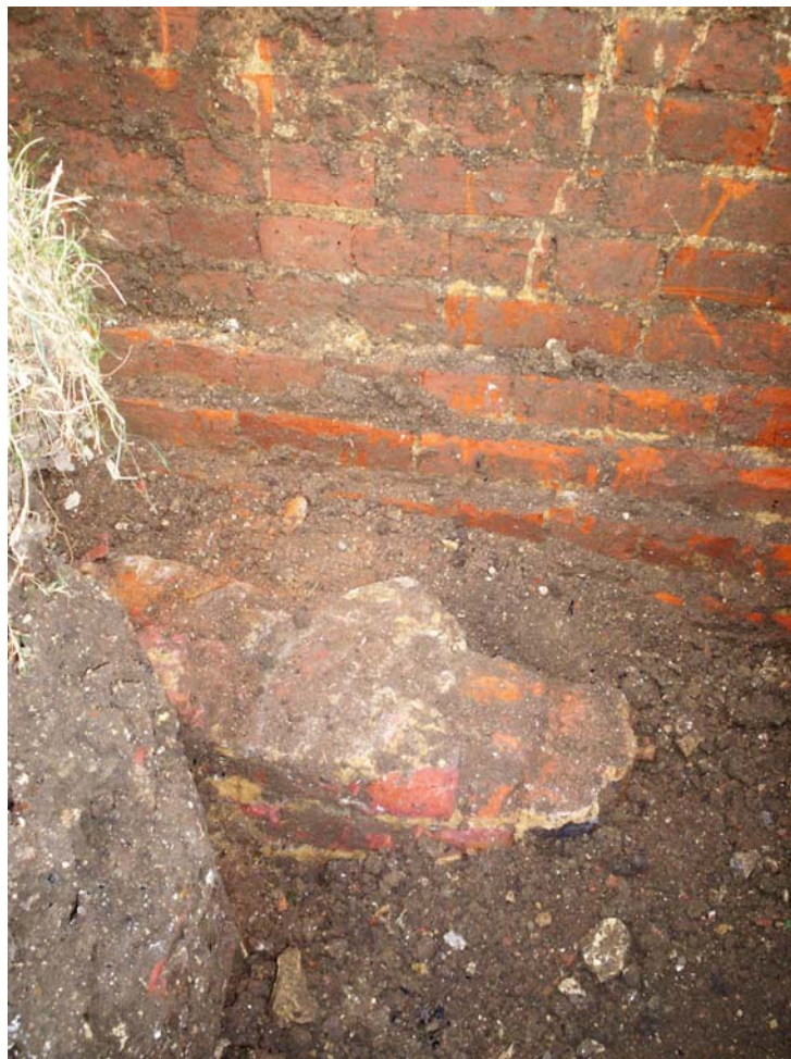
Plate 6. Stepped foundation of wall [04] and remains of 'wall' [2] in foreground; facing north-west.
