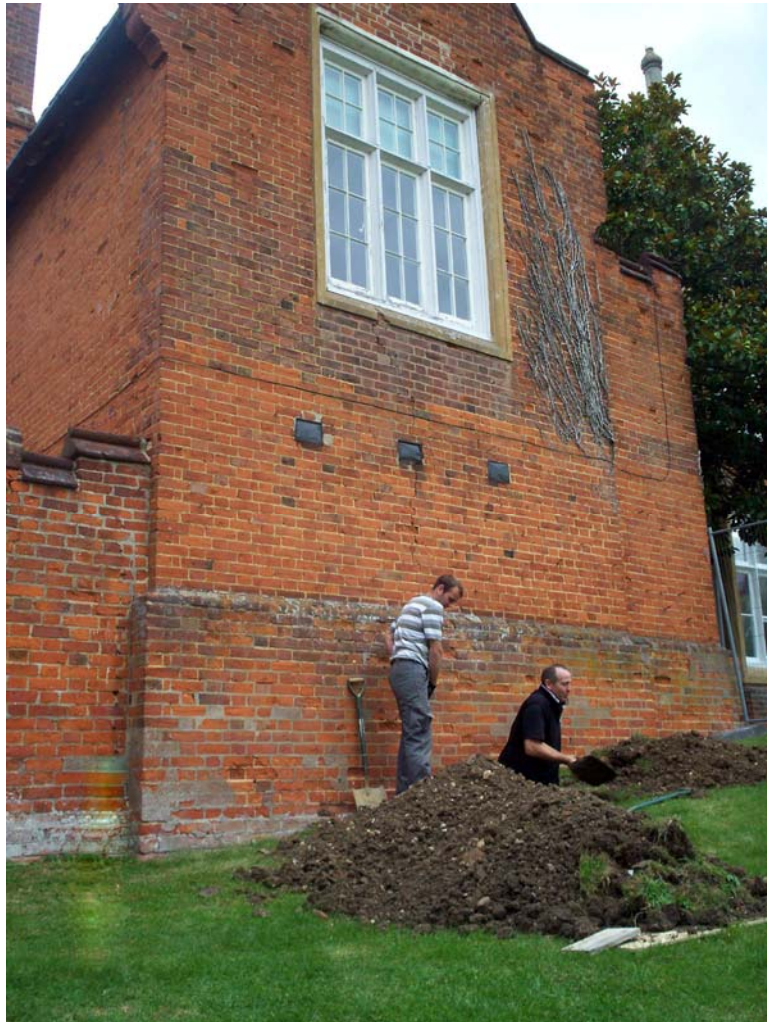
Plate 1. South-west facing elevation of 'kitchen' with test pit being excavated by staff of Brown and Ralph, facing east
