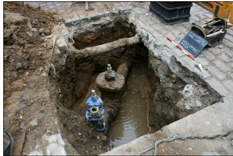
Plate 2. Looking south at fully excavated Contractor's trench, 0.50m scale
