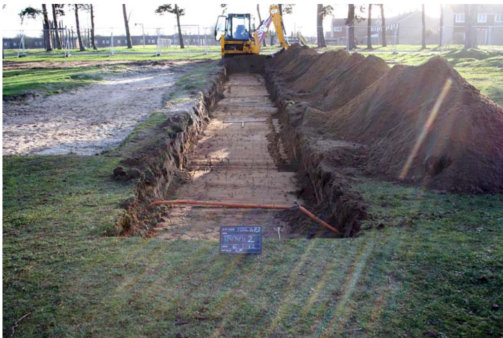
Plate 3. Trench 2, view from north end
