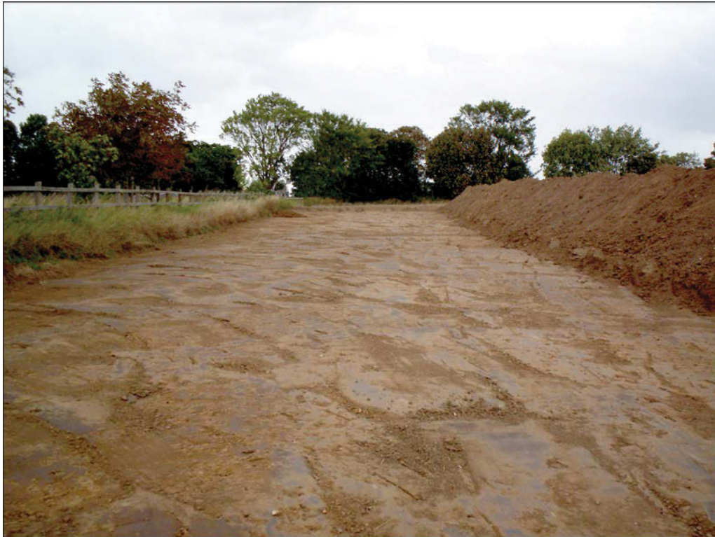
Plate 1. The easement strip, looking north
