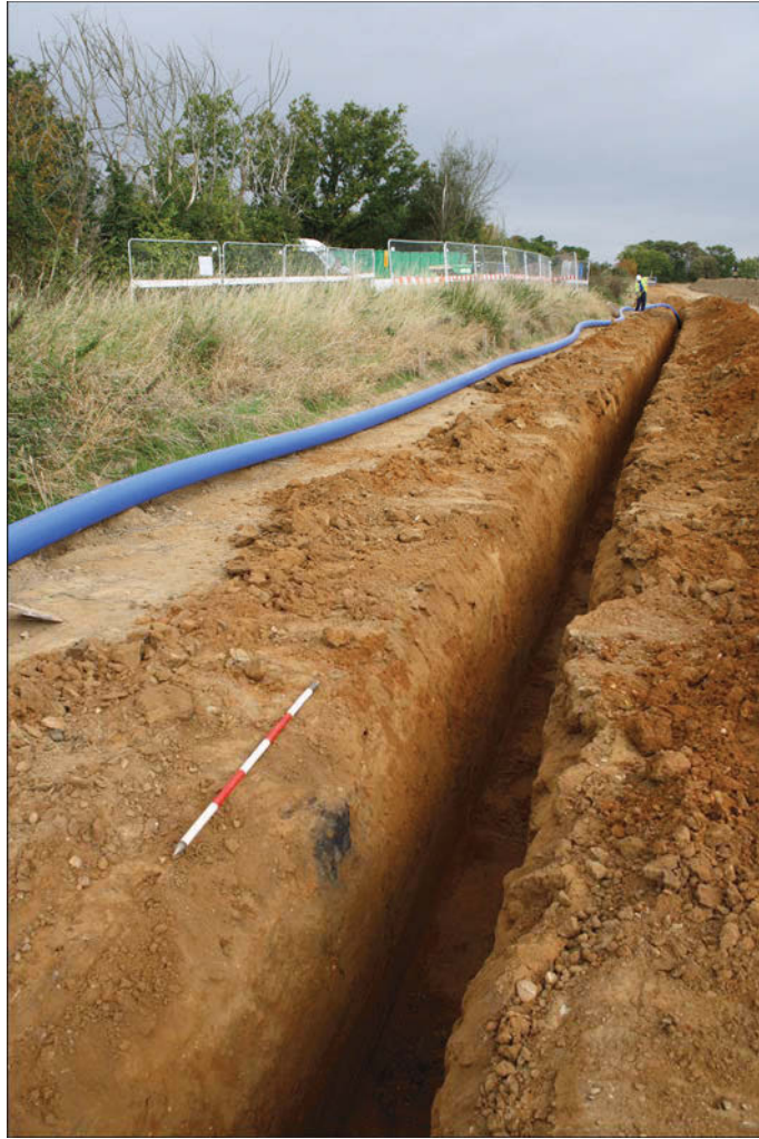
Plate 5. Pipe cut, looking north-west with pit [32] in the foreground
