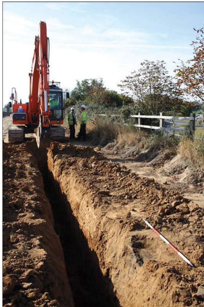
Plate 3. Machining the pipe cut with pit [30] in foreground, looking south-west
