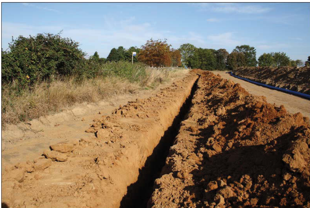
Plate 2. The pipe cut, looking north
