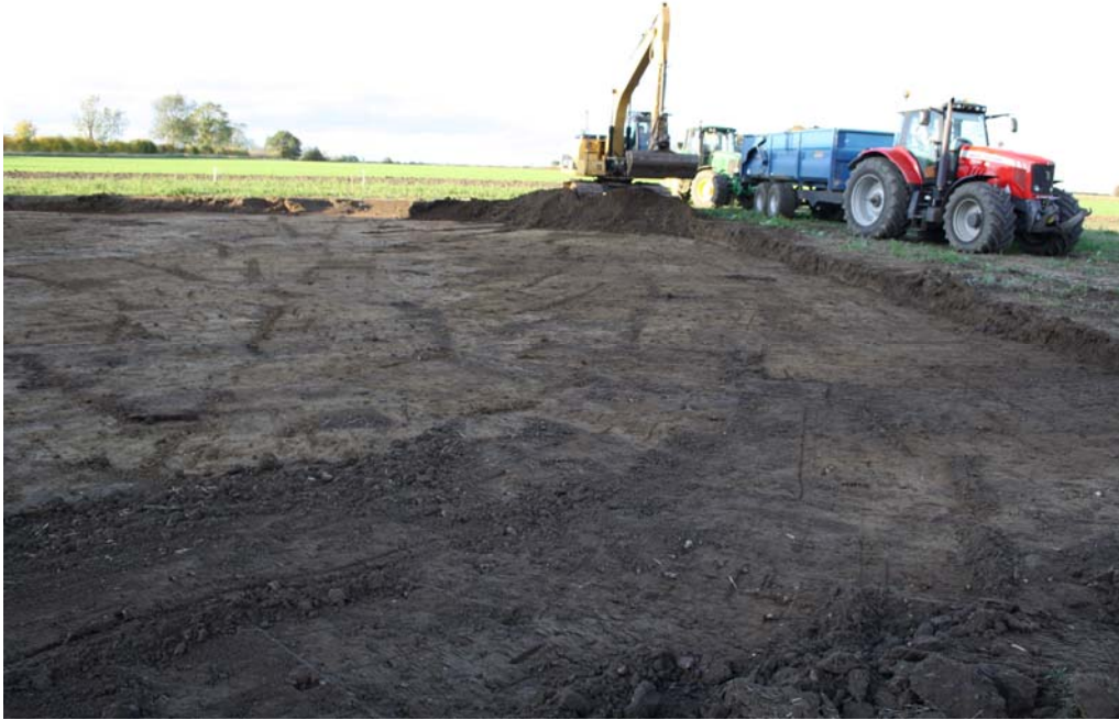
Plate 1. Stripping the topsoil from the site
