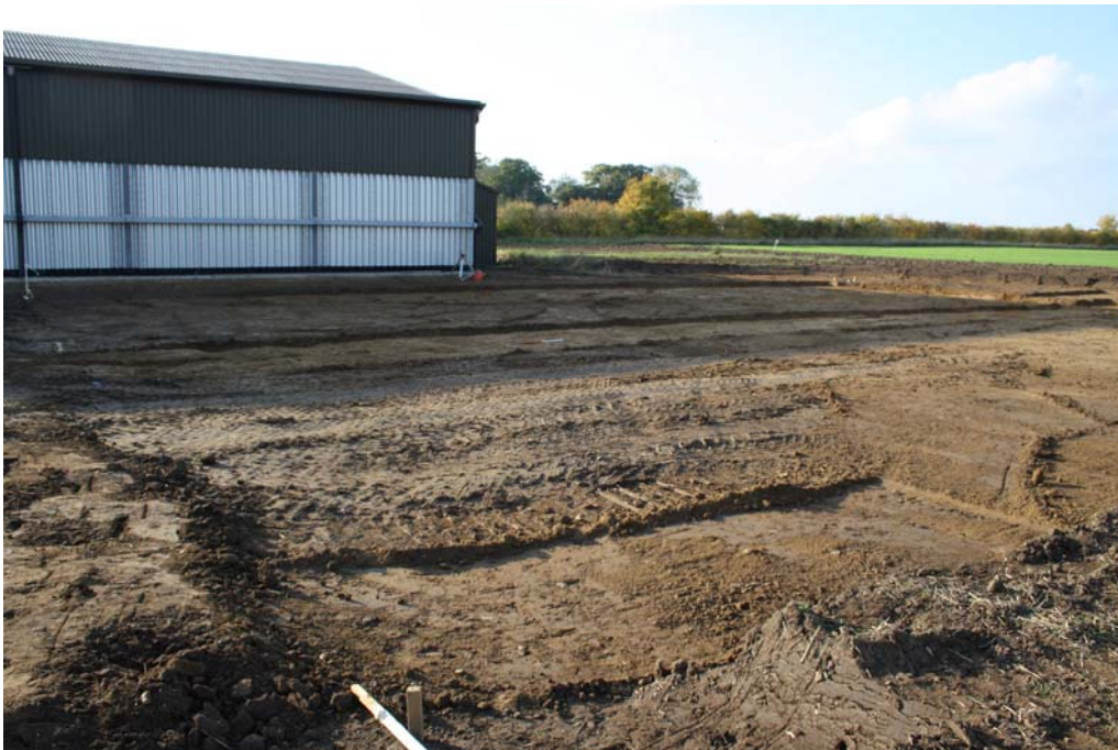
Plate 2. Levelling for groundworks looking south-west
