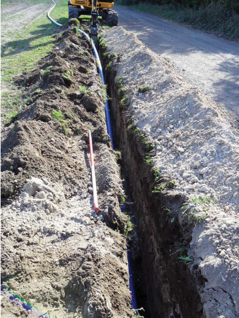
Plate 1. Pipe trench looking south-east
