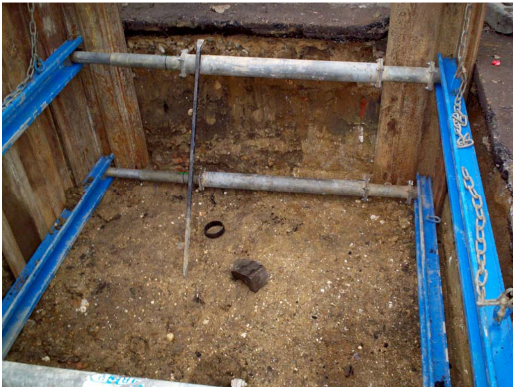
Plate 1. Manhole trench looking south, partially excavated
