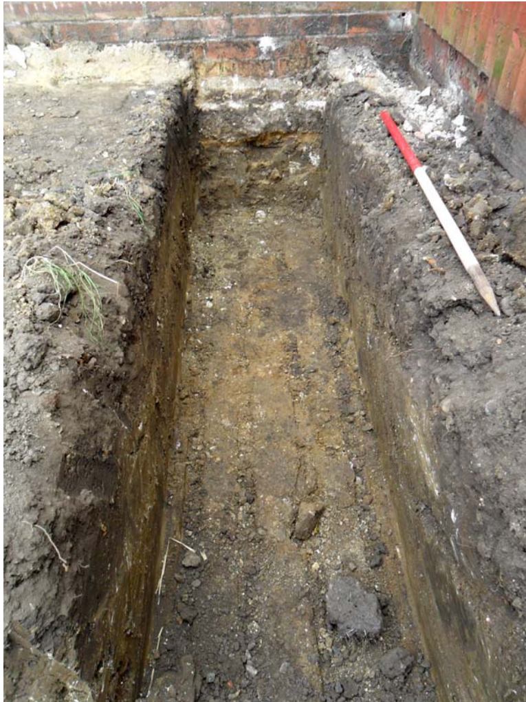
Plate 1. End of foundation trench for the new conservatory, looking east
