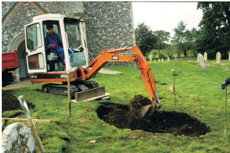
Plate 2. Excavation of the soakaway, looking south-west. C.Phillips
