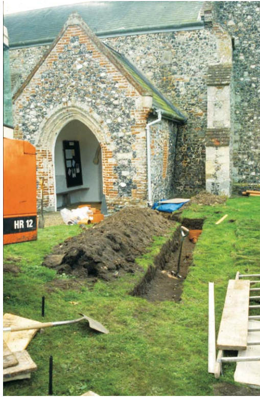
Plate 1. Excavation of the trenches, looking south. C.Phillips
