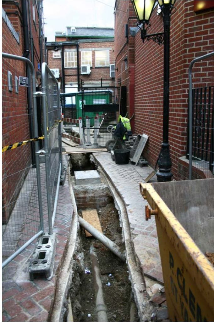
Plate 1. The service trenches to the south of the buildings, looking east
