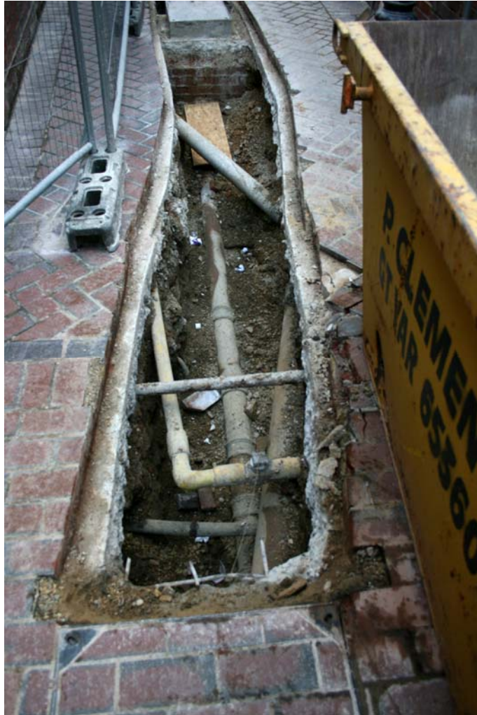
Plate 2. Detail of service trench to south of the buildings, looking east
