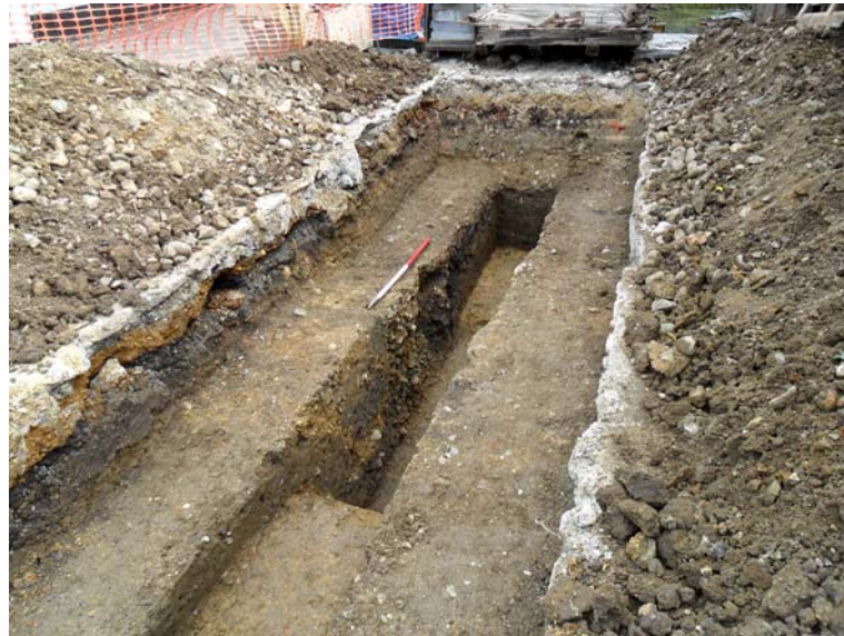
Plate 16. Trench 2, pit [20], looking north-east
