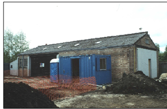
Plate 1. Garage workshop, perhaps dating to WWII
