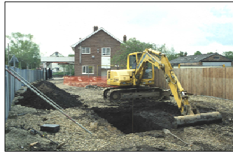
Plate 2. Machine excavation of Trench 3, looking south
