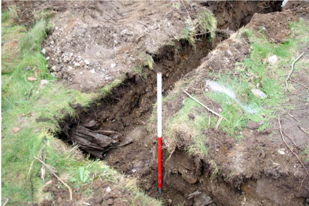
Plate 3. The south-west corner of the new foundation trenches showing modern soakaway
