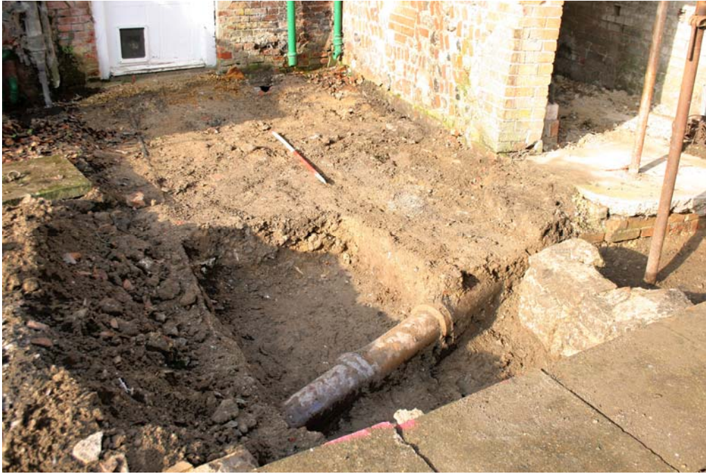
Plate 6. Evaluation area showing position of trench, looking west
