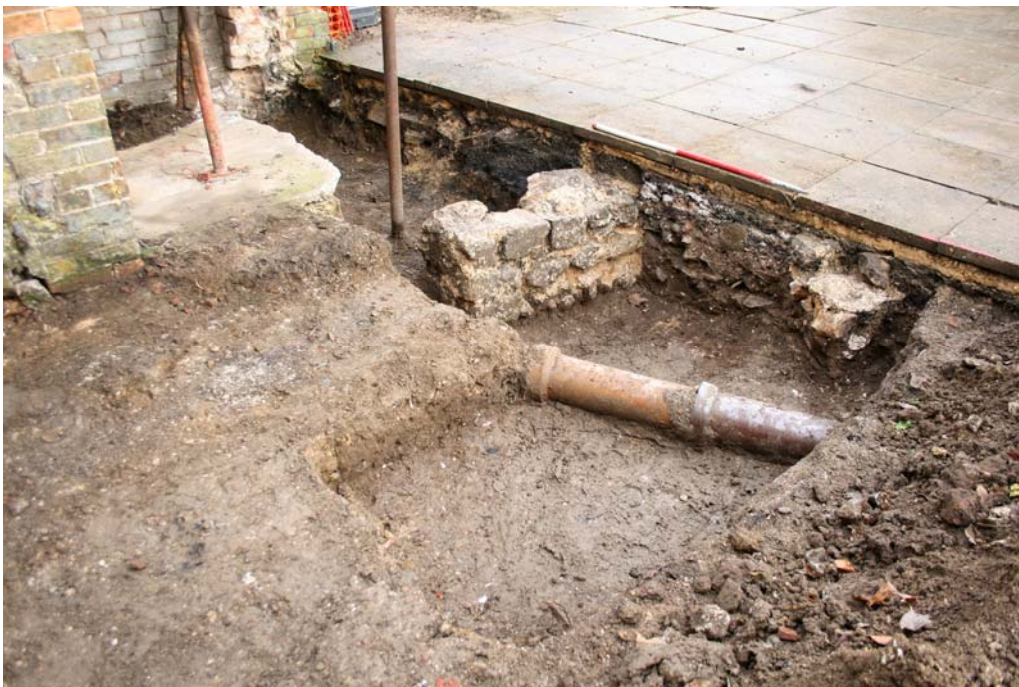
Plate 7. Evaluation area showing position of trench, looking north-east
