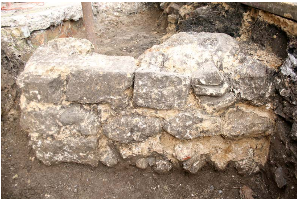
Plate 9. Close-up of wall [11], looking north
