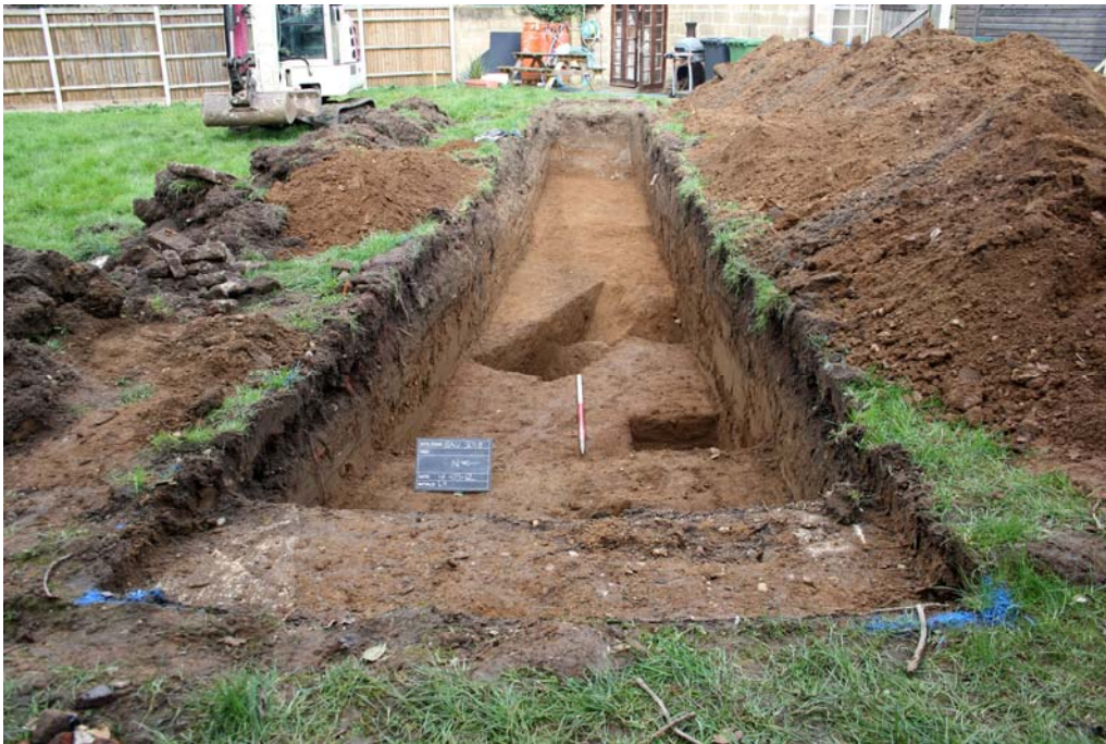
Plate 1. General view north-east along trench
