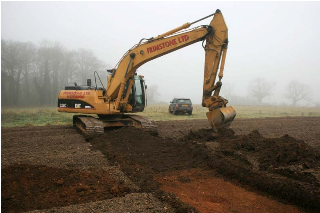
Plate 1. Machining looking south west
