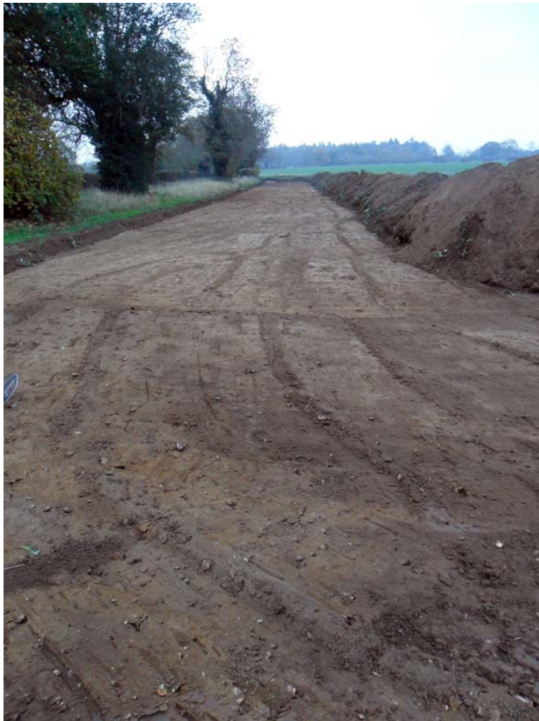
Plate 1. The stripped easement, showing subsoil layer (2)
