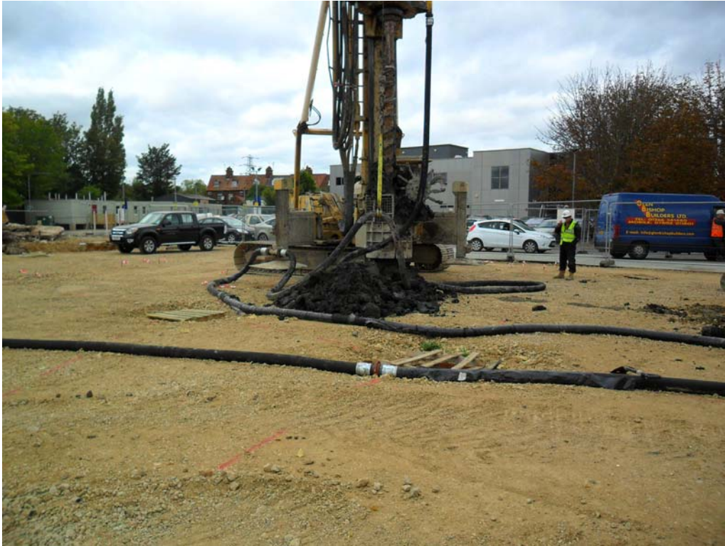
Plate 1. Piling in progress
