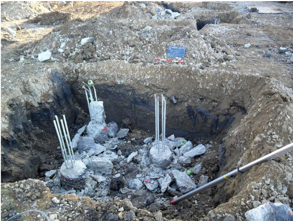
Plate 2. A typical stanchion pit hole
