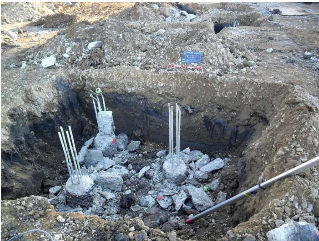
Plate 2. A typical stanchion pit hole
