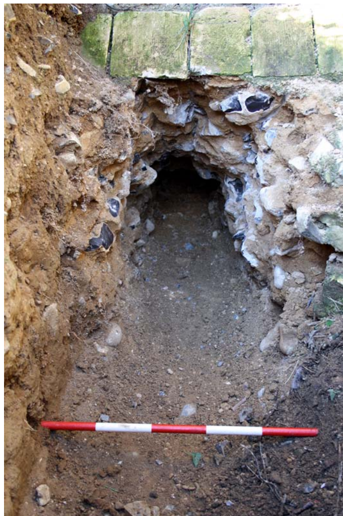
Plate 2. Hole drilled through church wall, facing north
