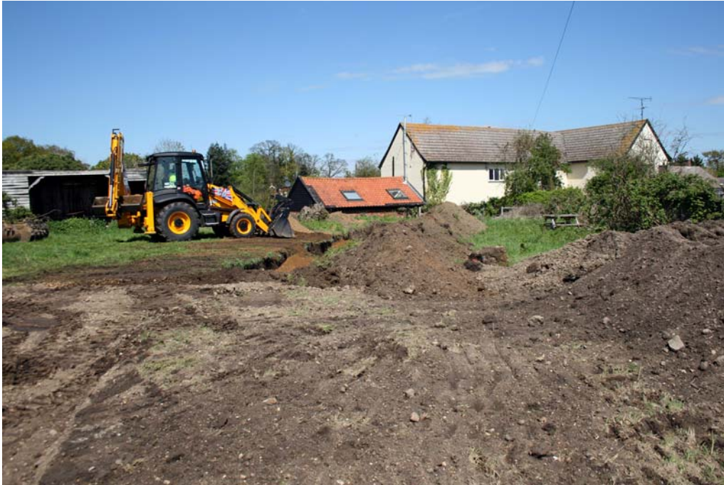
Plate 5. The site (during backfilling), looking north
