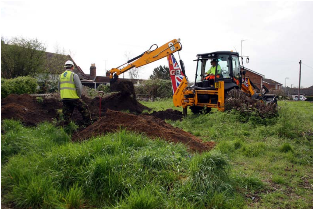
Plate 1. Machining, looking south
