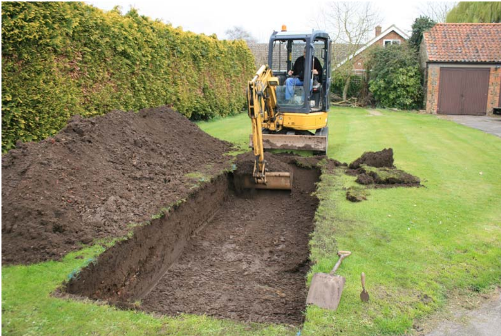
Plate 2. Machining (Trench 1), looking east
