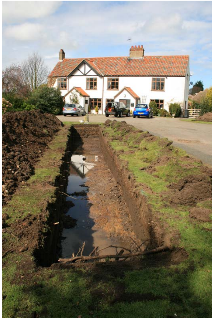
Plate 3. The site (Trench 2), looking north
