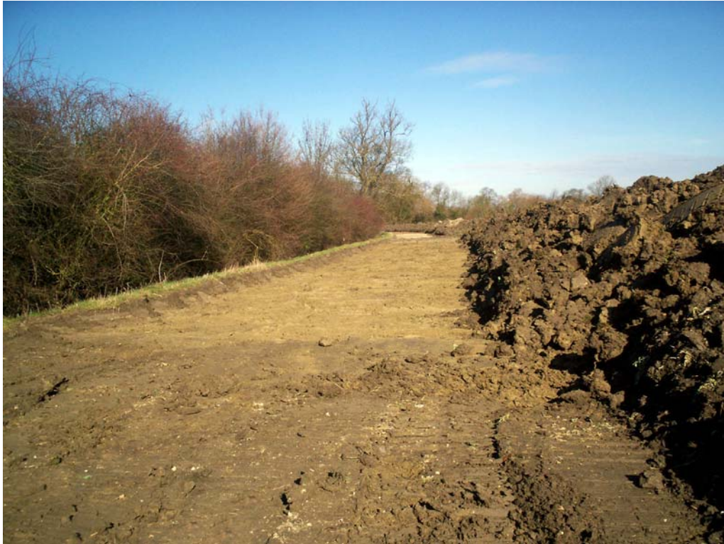
Plate 2. The easement between chainages 1600 and 1900, looking north
