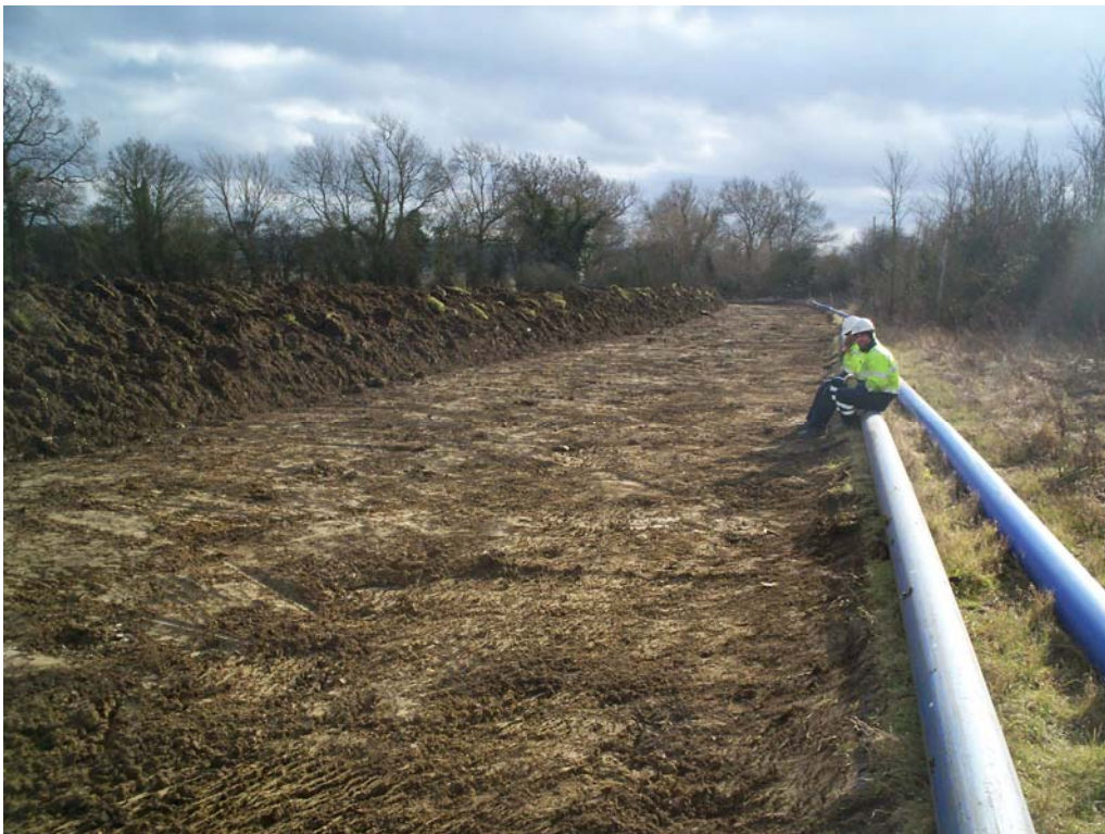
Plate 1. The easement between chainages 1500 and 1600, looking south
