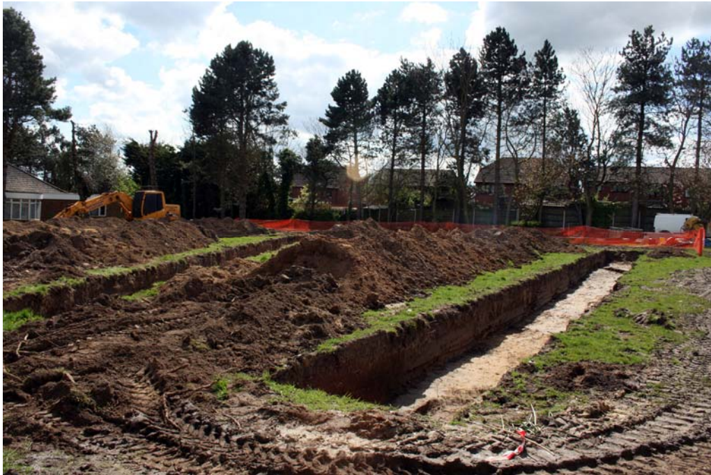
Plate 3. Trench 3, excavated ditches [52], [54], [56] looking east, 1m scale
