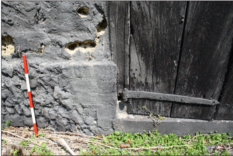
Plate 25. Close up of clay lump and low flint wall.
