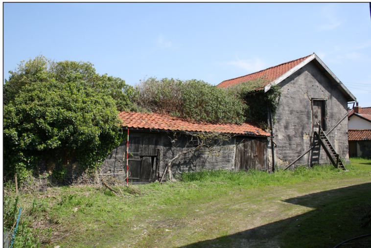
Plate 23. Whole southern elevation of the barn.
