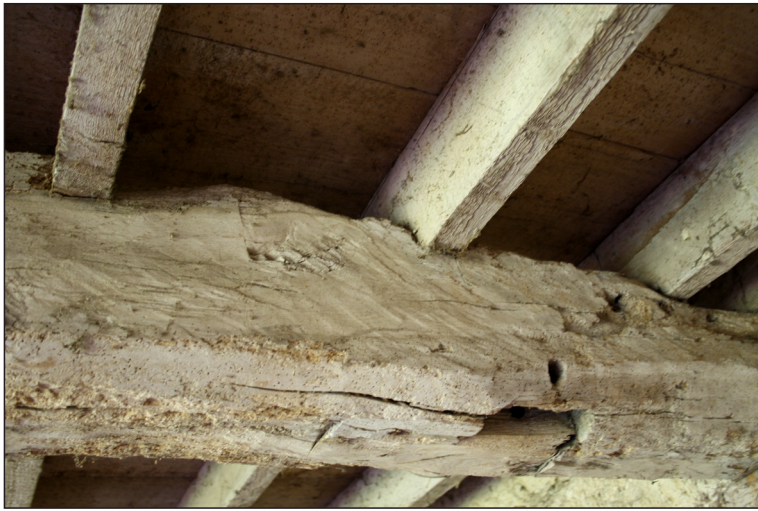
Plate 29. Evidence of axe and adze marks on the principal beam and posts.
