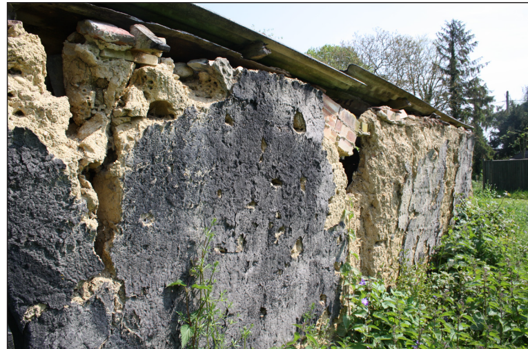
Plate 8. Close up of degraded small clay lump barn located just north of the barn.
