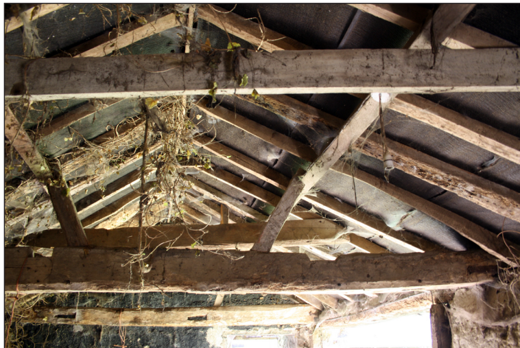
Plate 34. Cow shed roof structure.
