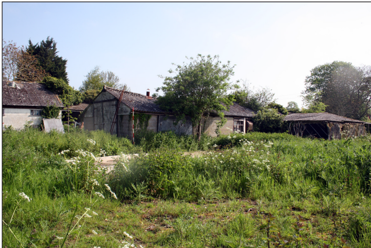
Plate 7. Looking north-east at further farm outbuildings north of the barn.
