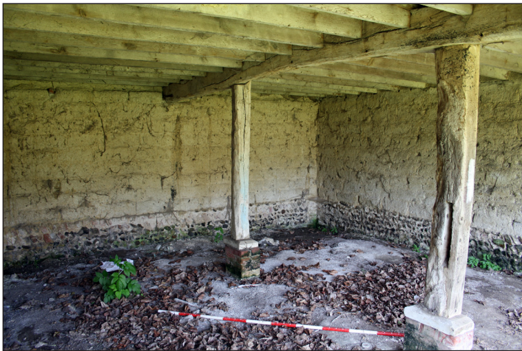
Plate 27. Interior of cart shed.
