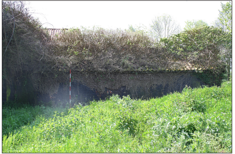
Plate 18. North elevation (rear) of cow shed.
