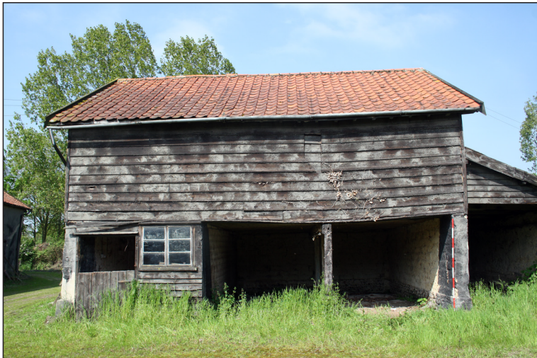
Plate 11. Front elevation of the barn showing weather boarding.
