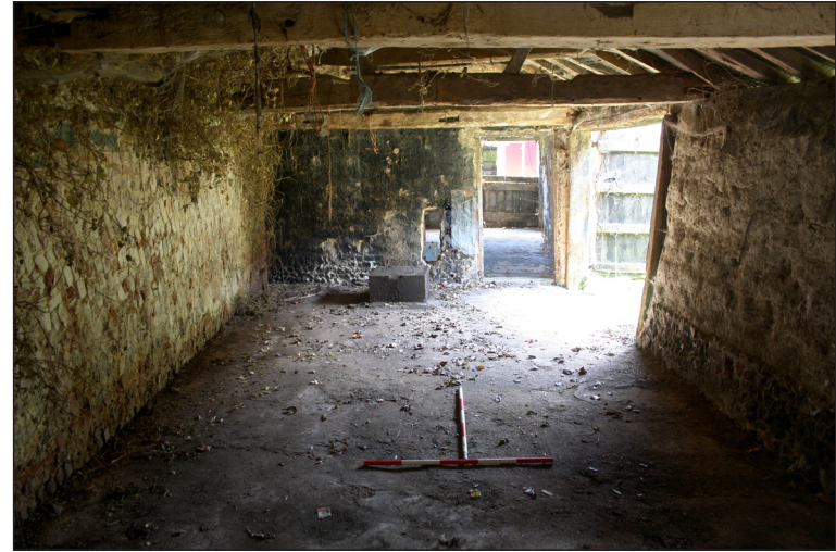
Plate 33. Interior of the cow shed. East facing.
