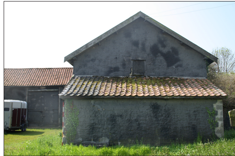
Plate 14. North elevation of the barn.
