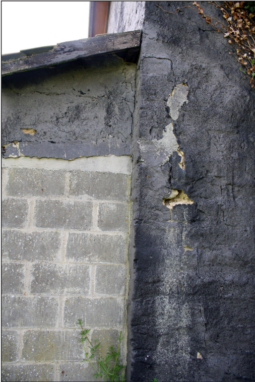
Plate 17. Close up of straight joint.
