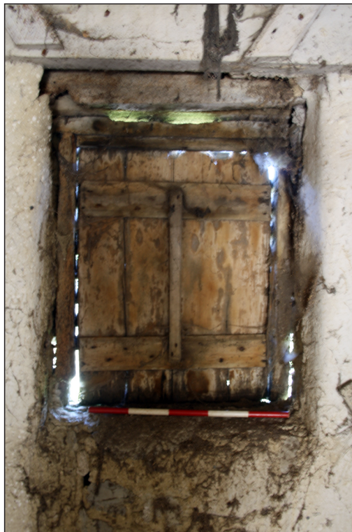
Plate 46. Interior view of possible airing window.
