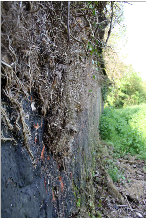
Plate 19. Looking along the north wall of the cow shed.
