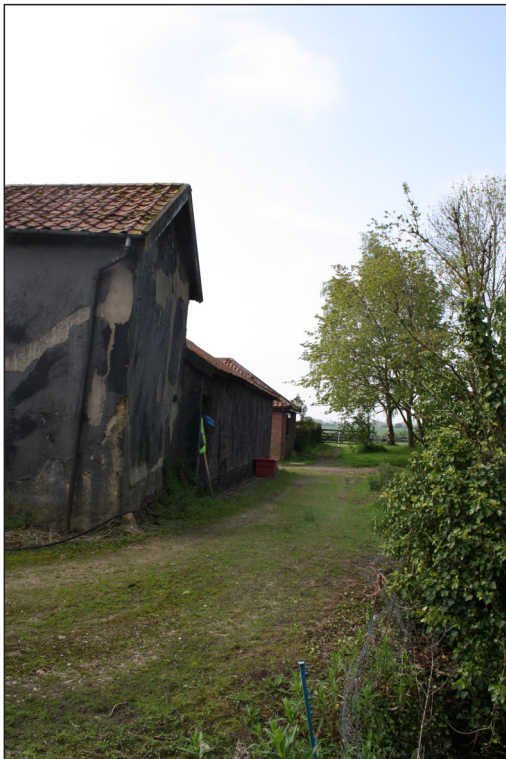
Plate 3. Church Farm barn. Facing south-south-east.
