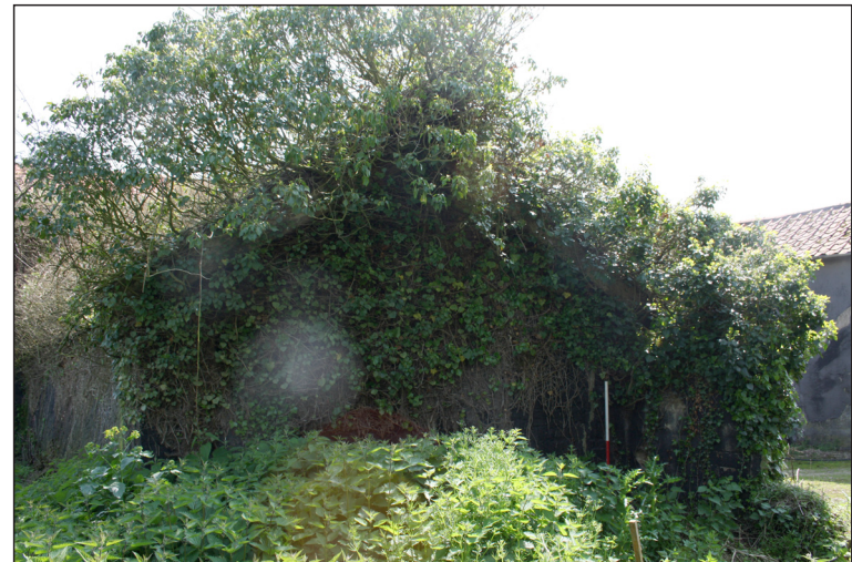
Plate 24. West elevation of cow shed.
