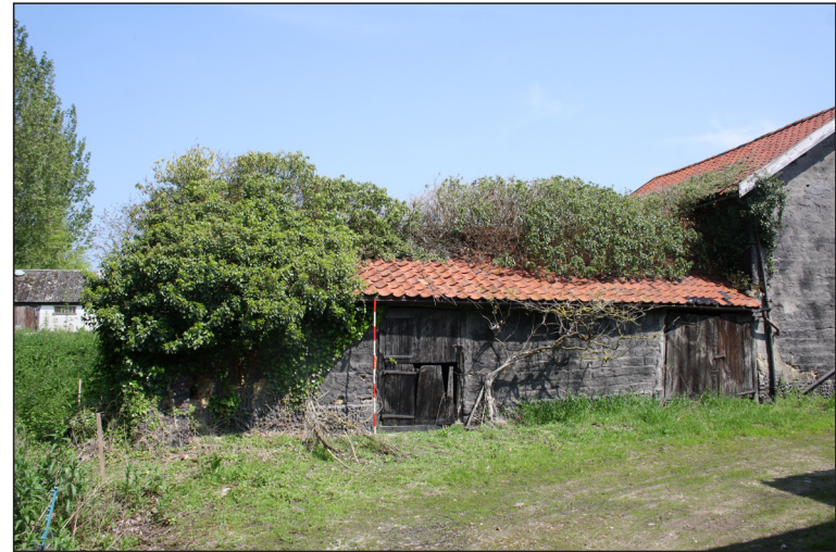
Plate 22. Southern elevation of cow shed.
