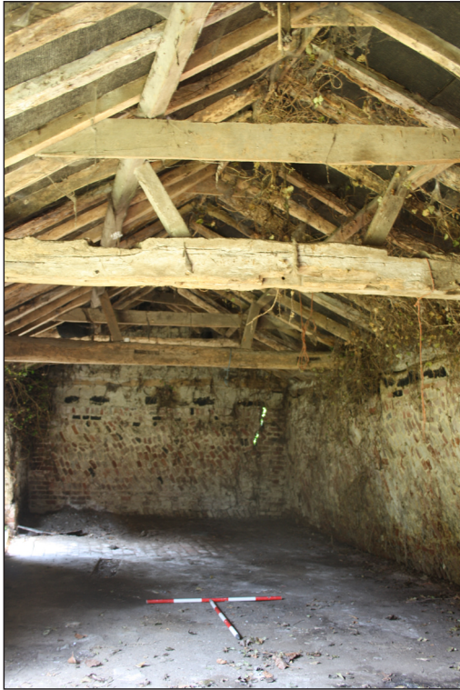
Plate 32. Interior of the cow shed. West facing.
