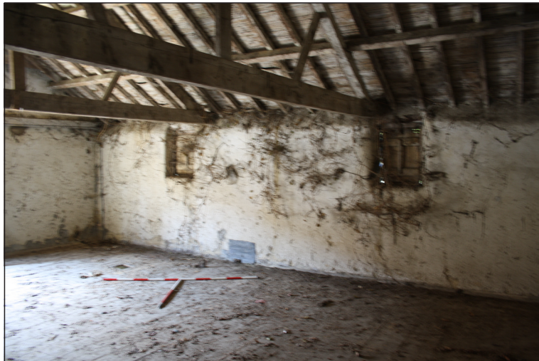
Plate 38. Hayloft interior. South-west facing.
