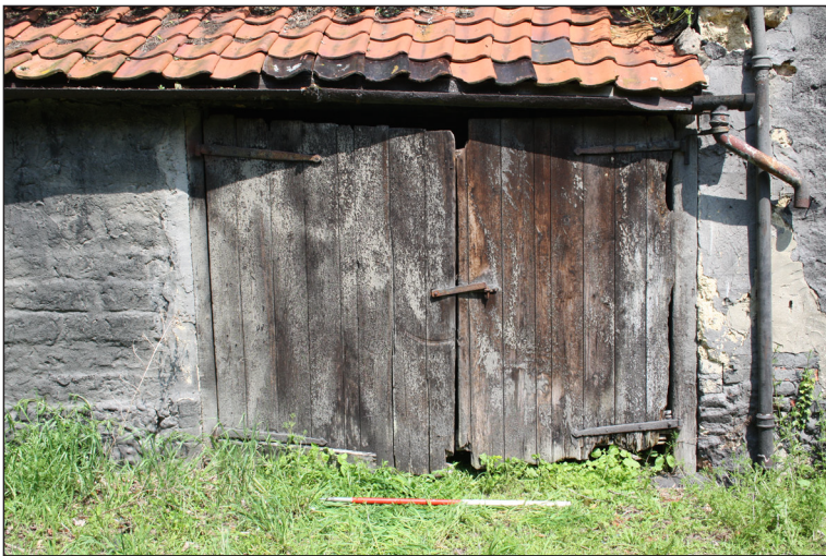
Plate 42. East door of cow shed.
