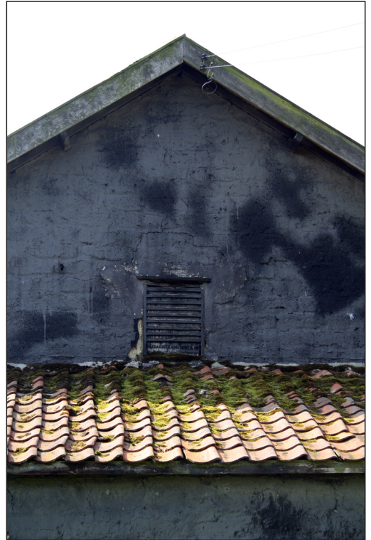
Plate 45. Exterior view of airing window.
