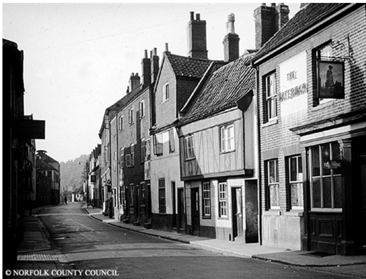
Frontispiece 1. King Street with the Waterman Public House and No. 144 beyond (Copyright Norfolk Count Council)
