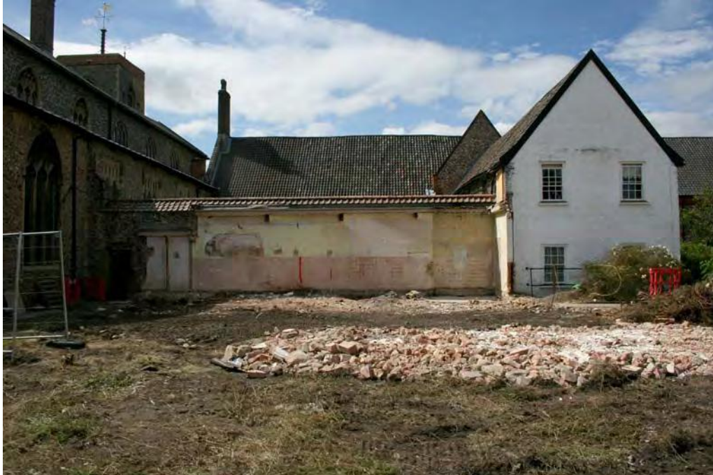
Plate 8. Watching Brief, demolished laundry block, looking west
