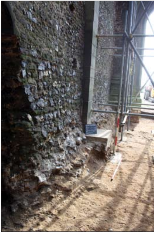
Plate 25. East internal wall of Gateway
