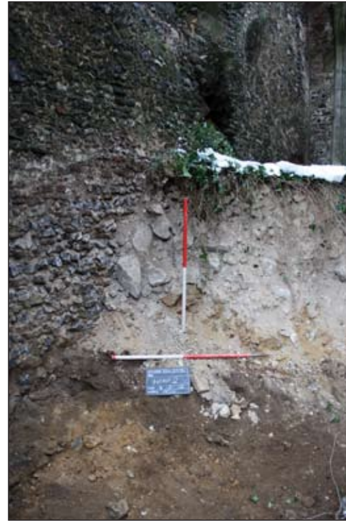
Plate 14. Cross section of collapsed wall
