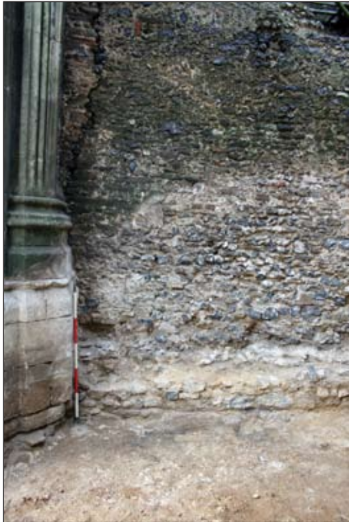
Plate 21. Main Gateway, post excavation
