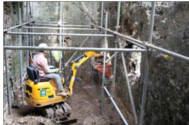
Plate 8. Machine excavation West Room
