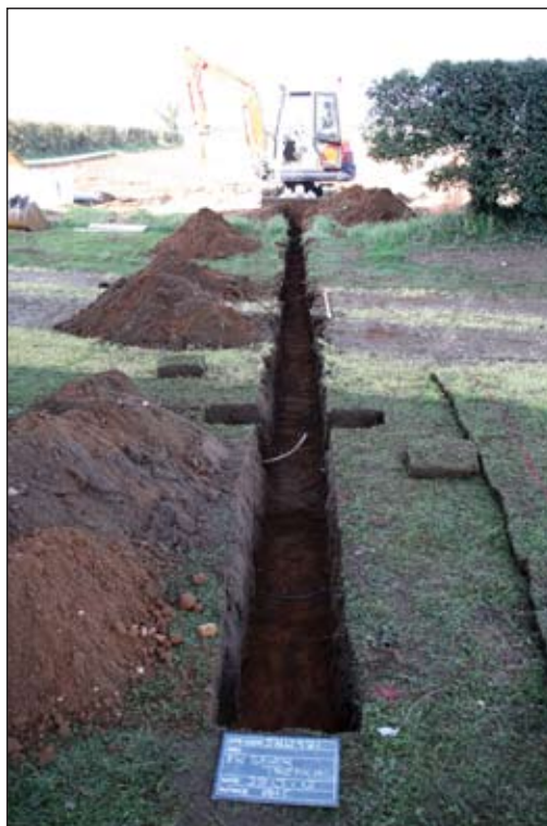
Plate 38. Plate 38. East-west sewer trench
