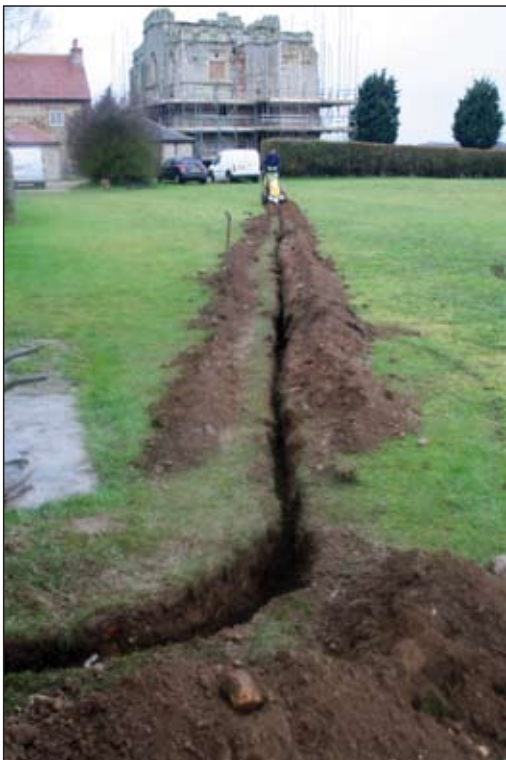
Plate 27. Electrical trench being dug towards the gatehouse
