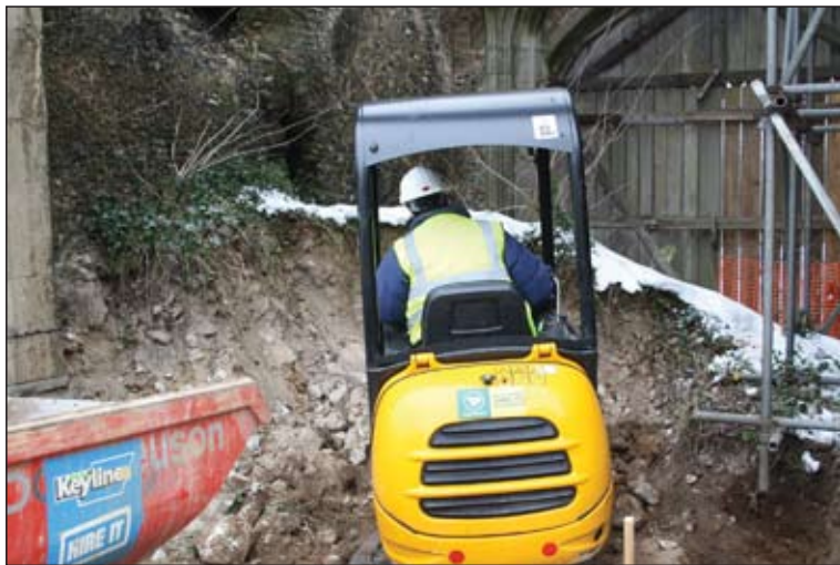
Plate 7. Machine excavation Gateway
