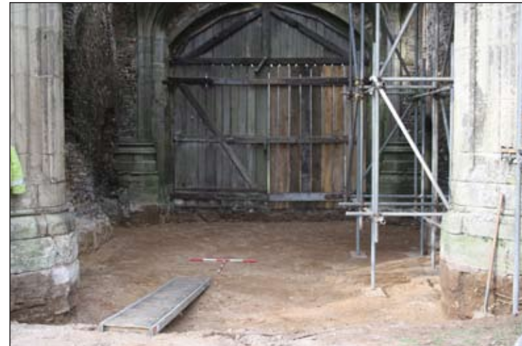
Plate 20. Main Gateway, post excavation
