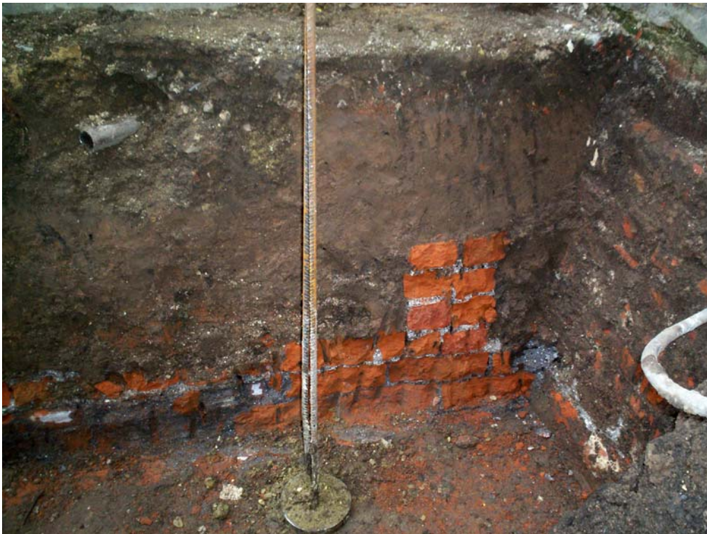
Plate 1. The north-western end of the ring beam showing structure {5} and the foundations of 3, The Crescent.
