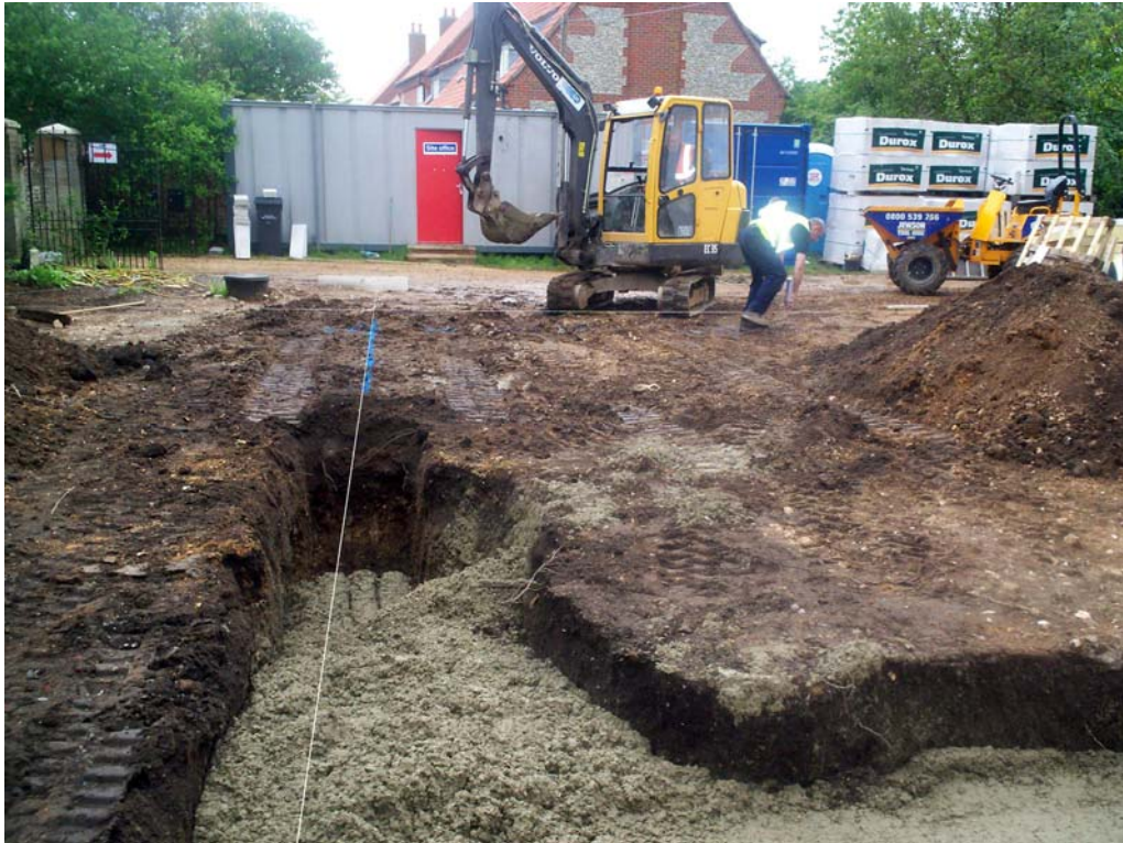
Plate 1. Orangery foundations under excavation, facing west
