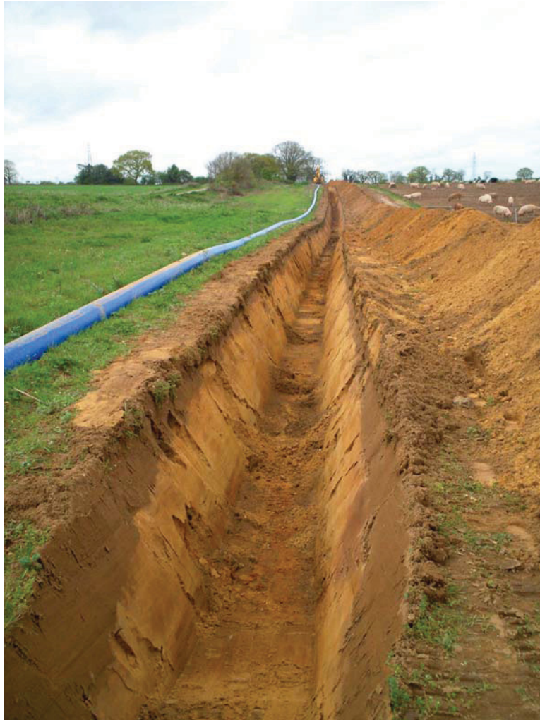
Plate 3. The pipe trench facing north-west
