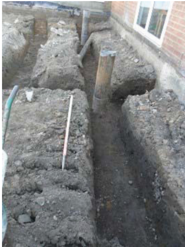
Plate 1. Excavated trenches and surface conditions
