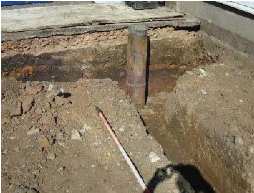
Plate 2. Overburden and subsoil in trenches
