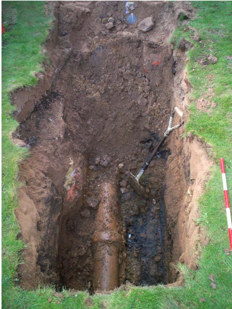
Plate 1. The manhole trench facing west, with foundation {4} exposed on the left
