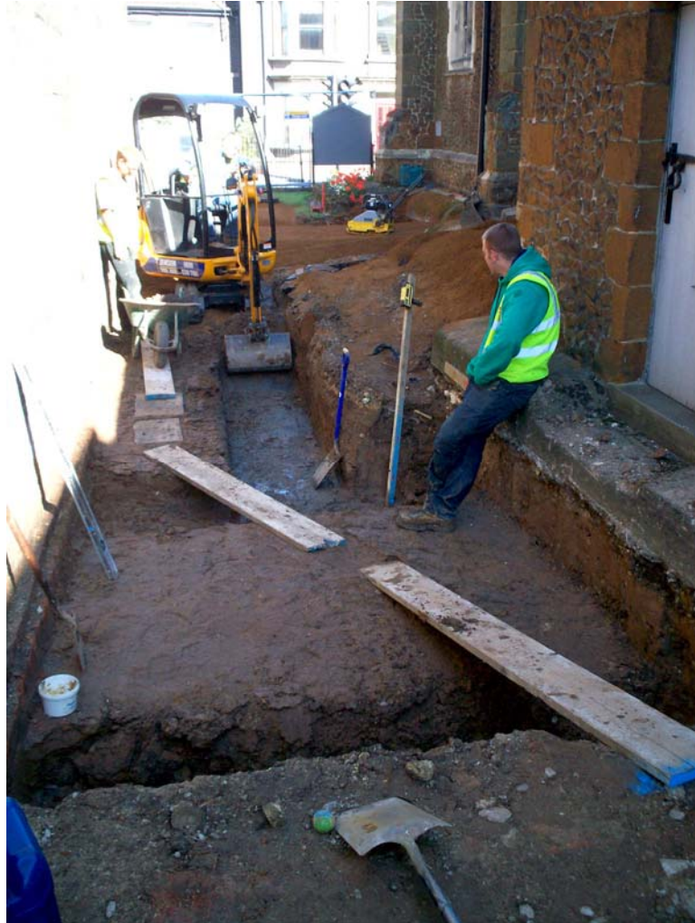
Plate 2. The foundations under excavation, facing east
