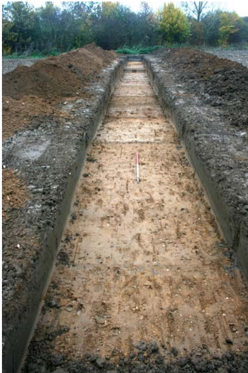
Trench 03, looking north-east
