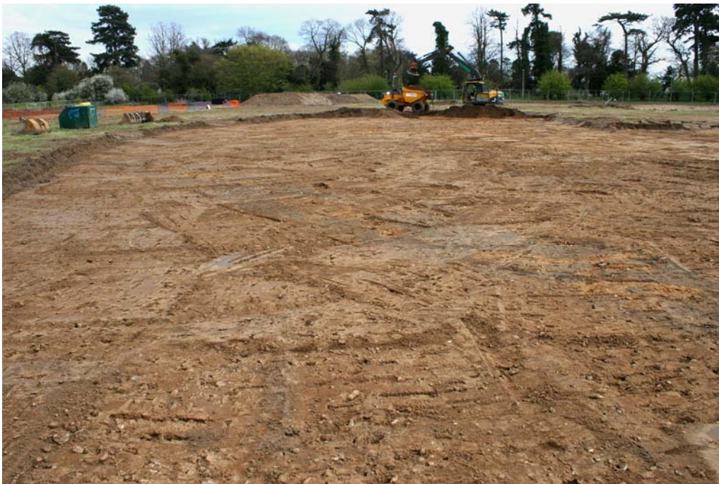
Plate 2. Stripping of the school footprint, looking north-east
