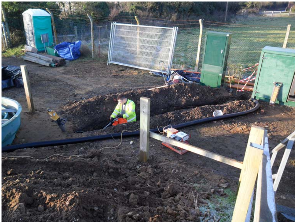
Plate 3. The trench across the access track, facing north-west
