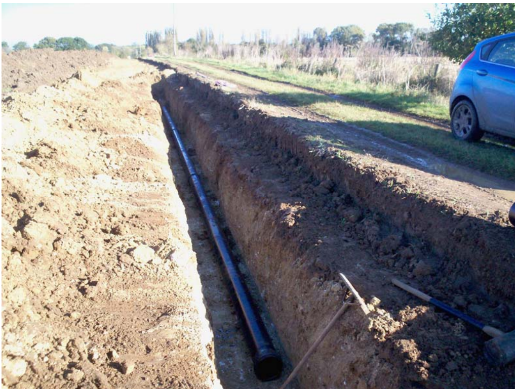
Plate 1. Cable trench and easement, facing north-east
