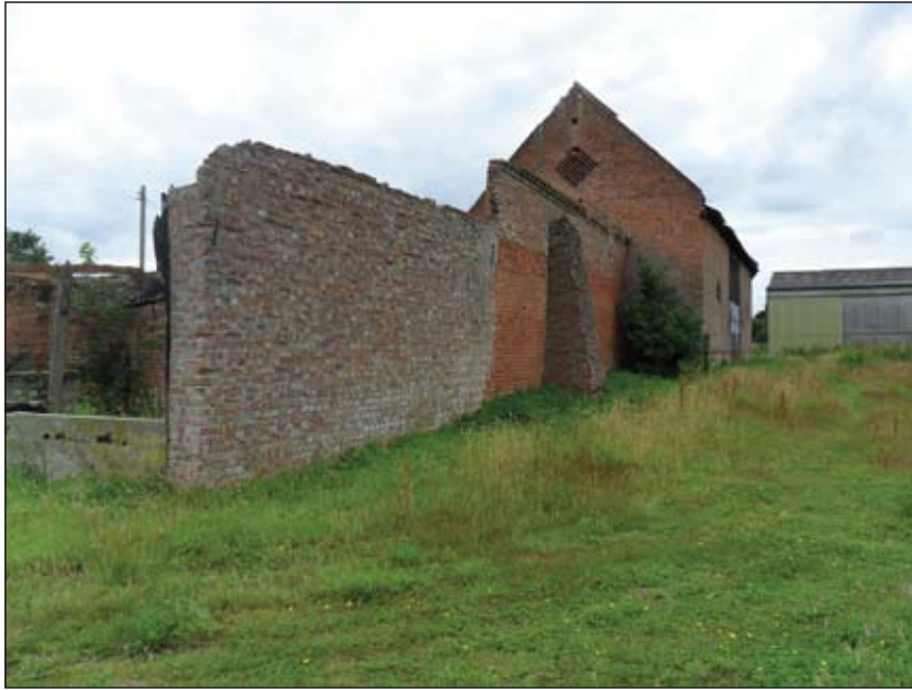
P9. East wing B, side wing and main barn, looking south
