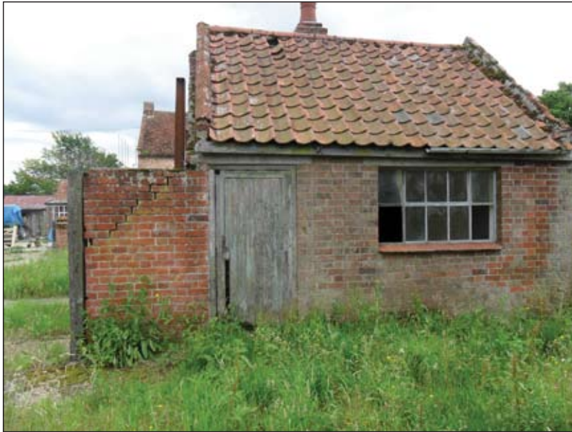
P17. Garden shed, north-western elevation, looking south-east
