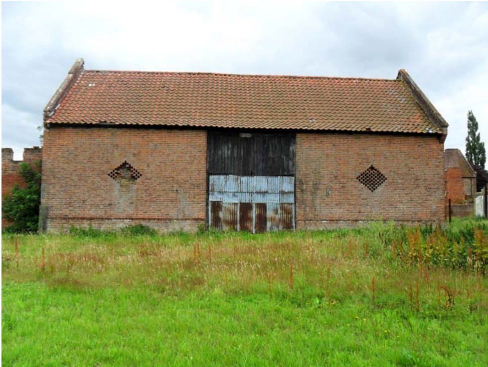
Plate 3. North-western elevation of main barn, looking south (Fig 5 P13)
