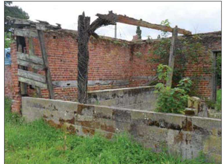
P6. East wing B, showing shell of timber framing, looking south
