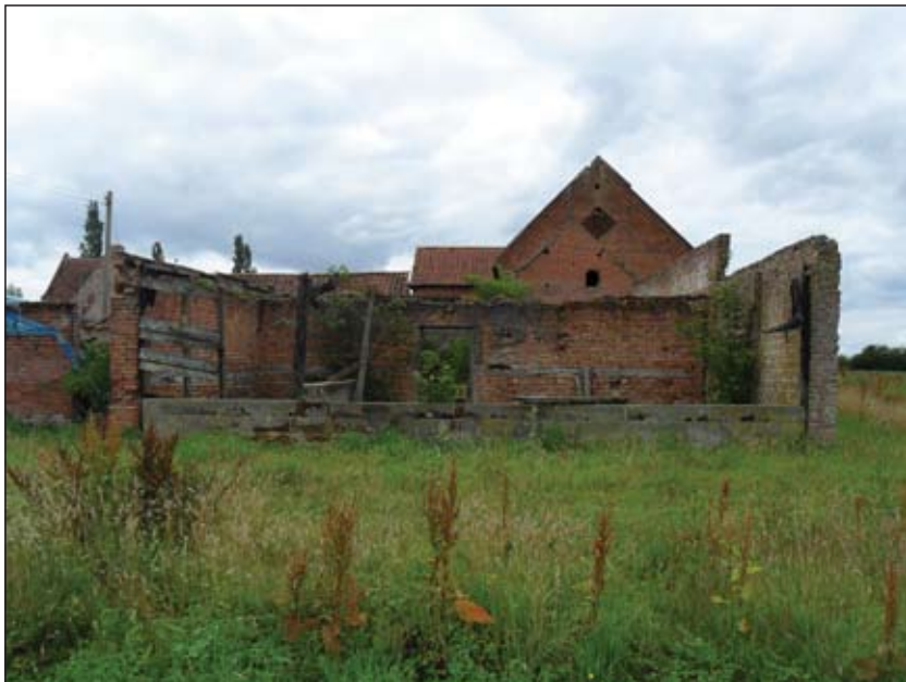
P3. East wing B, looking south-west
