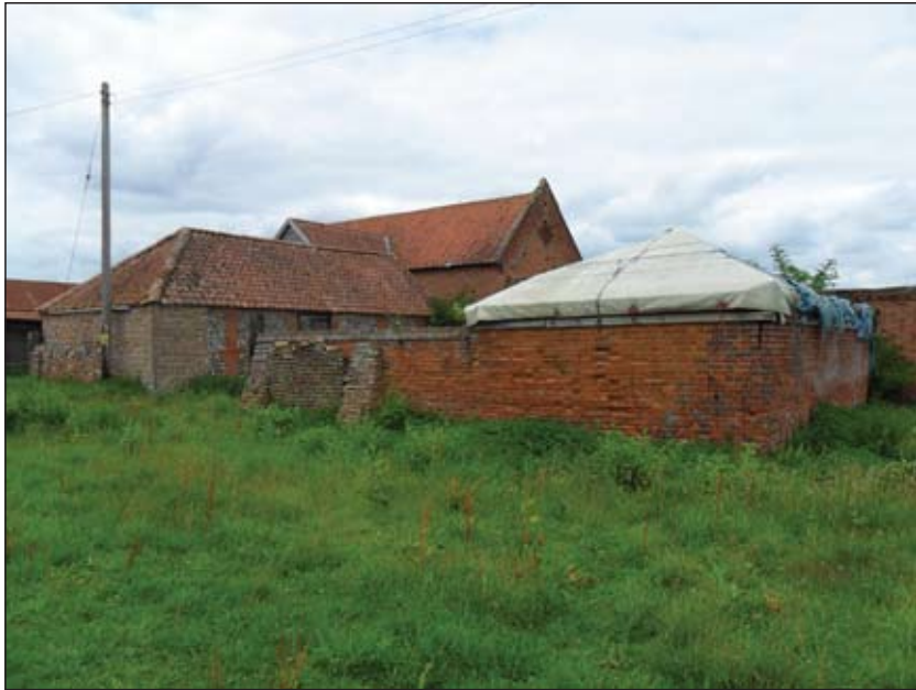
P1. East wing A, looking west
