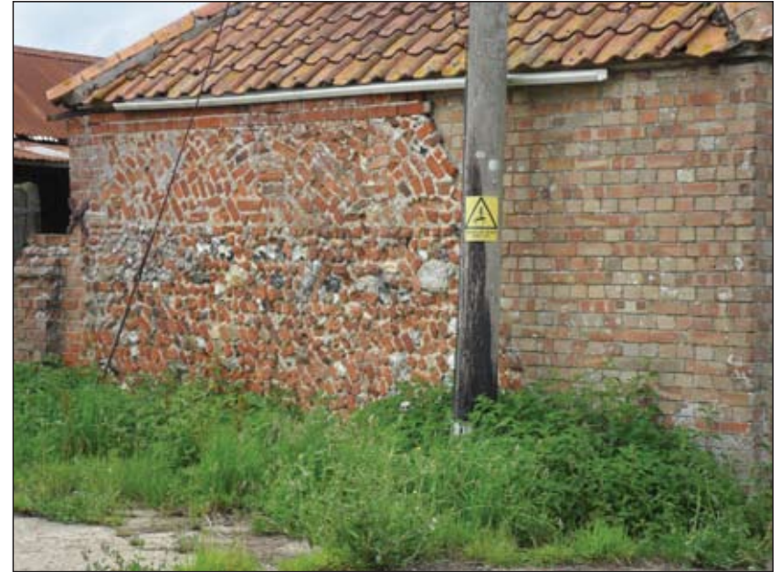
P33. South-eastern elevation of middle wing, looking west
