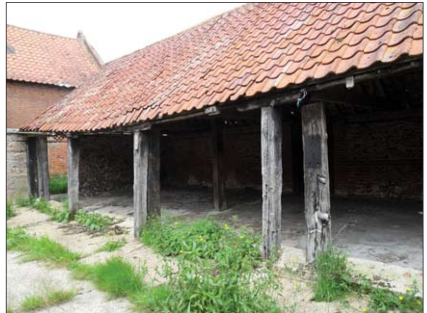
P24. Middle wing, looking north
