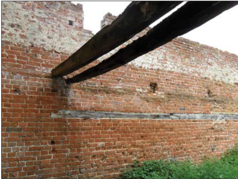
P27. Inside side wing, showing timber-framing, looking north-north-west
