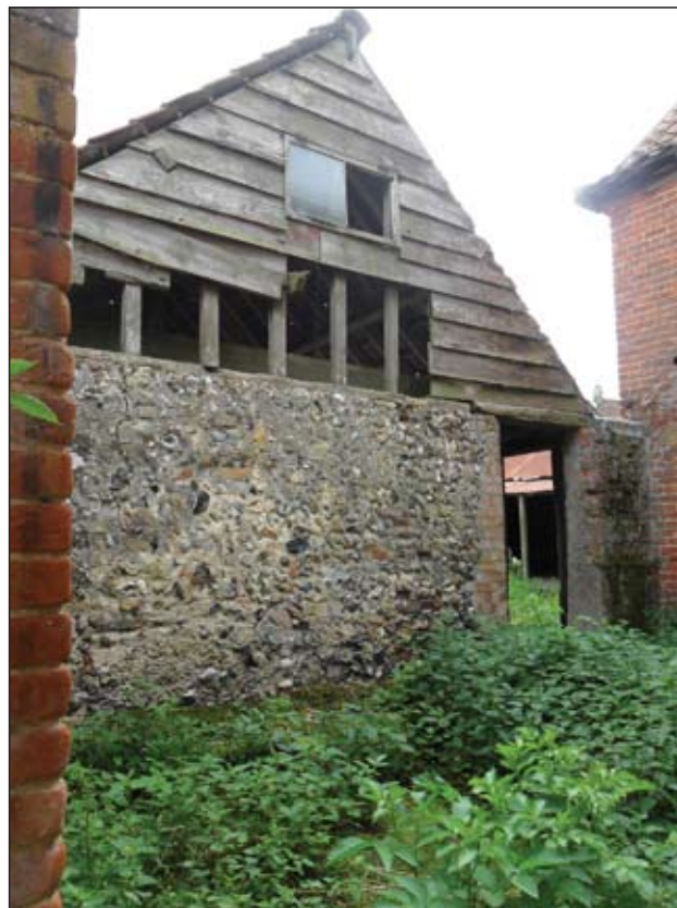
P31. North-eastern elevation of middle wing, looking south
