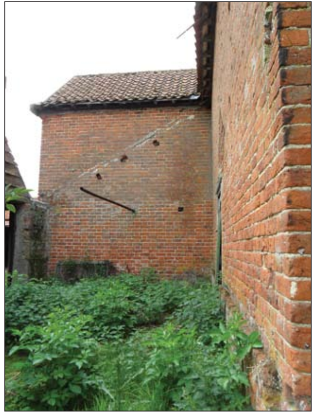
P30. South-eastern side of main barn porch, showing traces of lean-to, looking south-west
