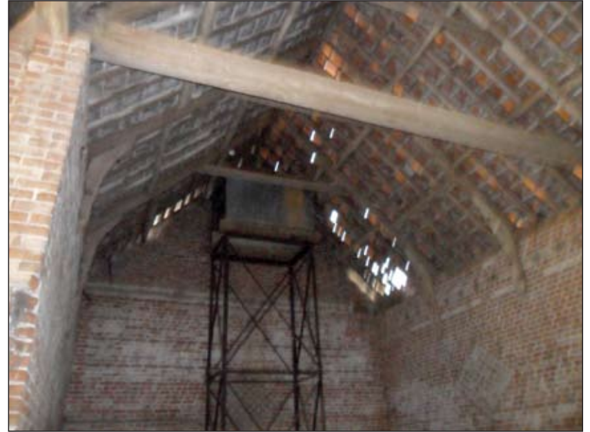
P26. Inside main barn, showing water tank and beams, looking west
