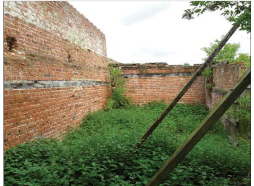
P28. Inside side wing, showing timber-framing, looking north-north-east
