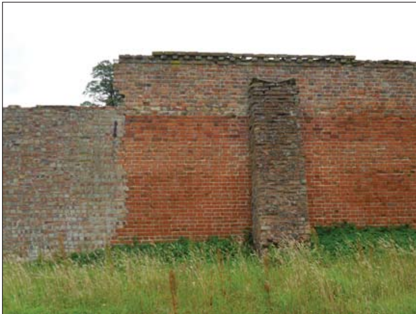
P11. Modern buttress and junction between east wing B and side wing, looking south-east
