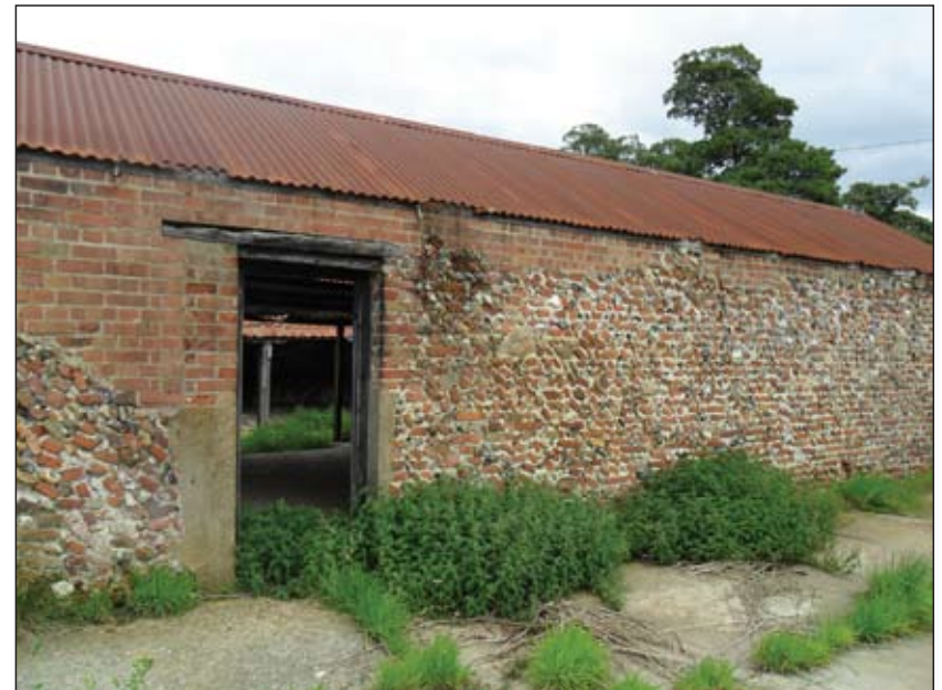
P20. West wing, showing doorway, looking east
