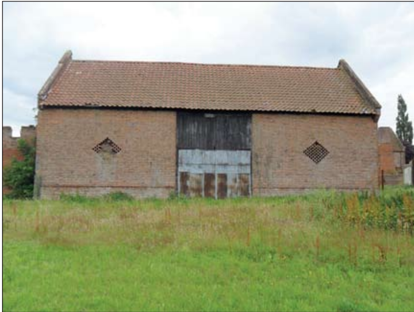
P13. North-western elevation of main barn, looking south-east
