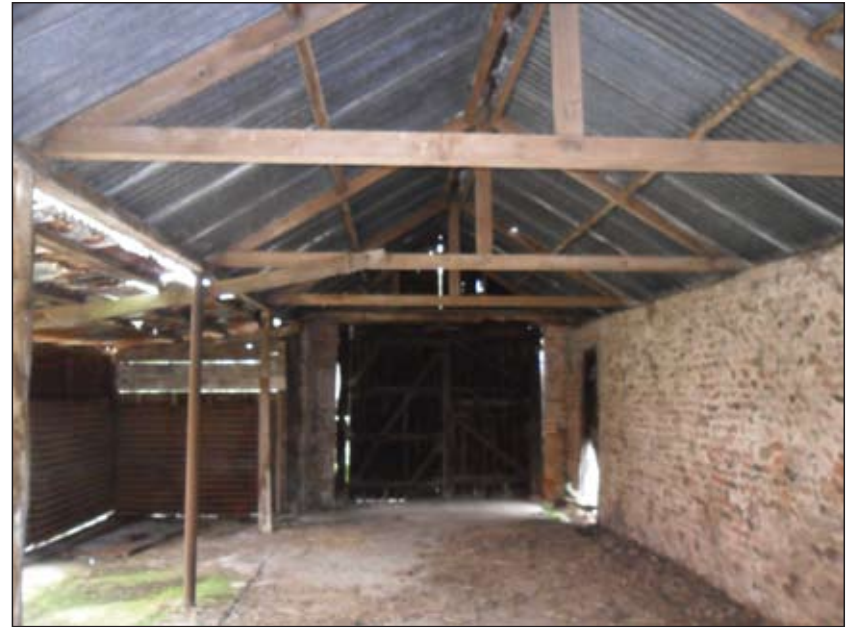
P22. Inside west wing, looking south-east
