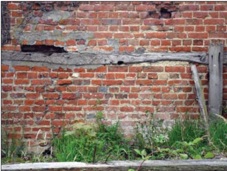
P5. Timber-framing within east wing B, looking south-west
