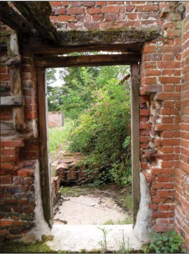
P29. Inside side wing, showing doorway leading to yard, looking south-east
