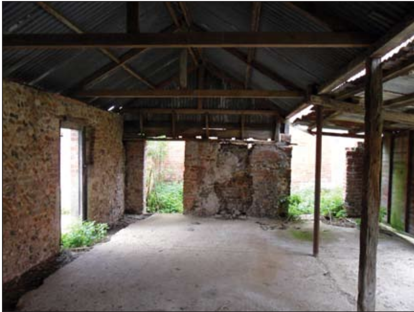
P21. Inside west wing, looking north-west
