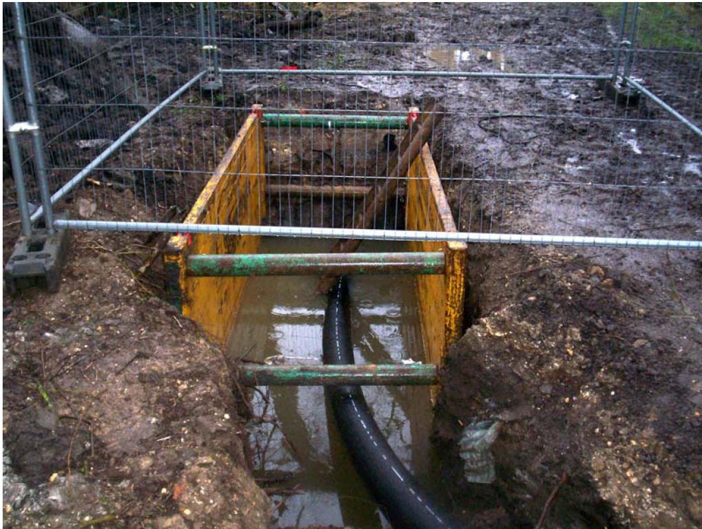
Plate 4. Drill Pit 4 facing north-east
