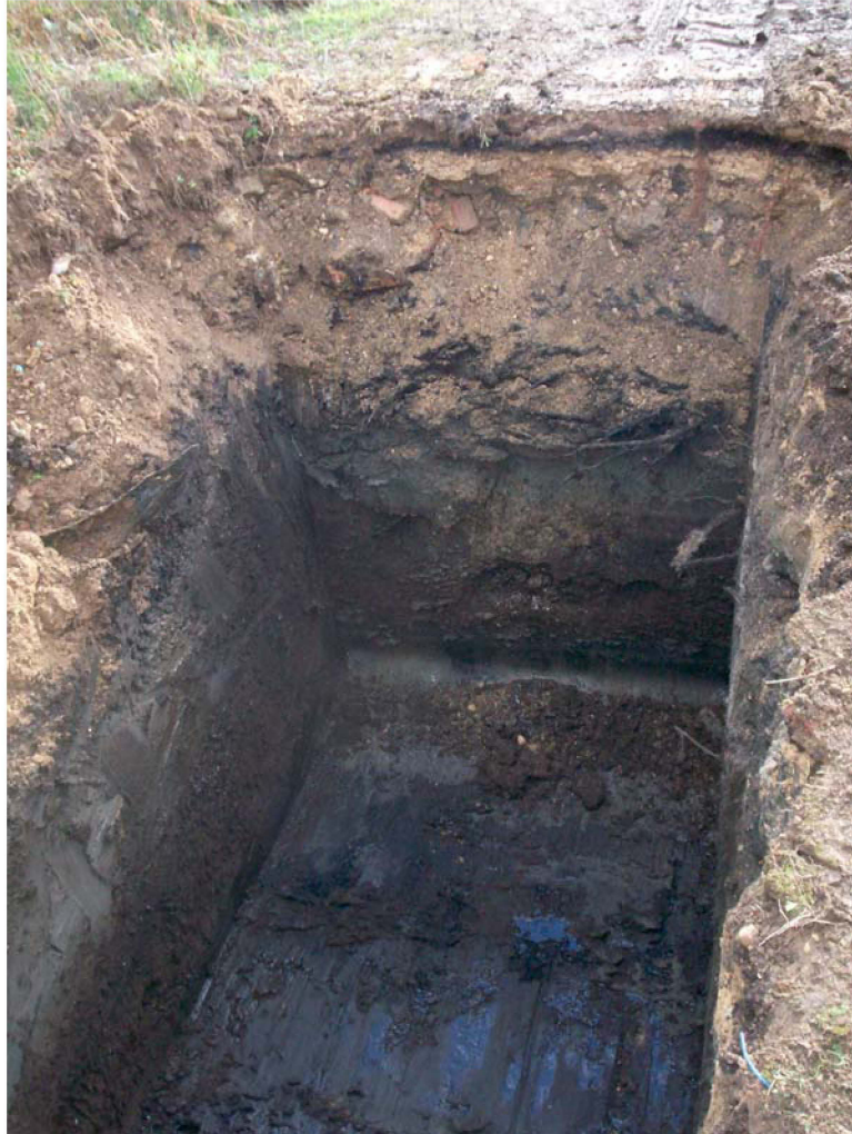
Plate 3. Drill Pit DP3 facing south
