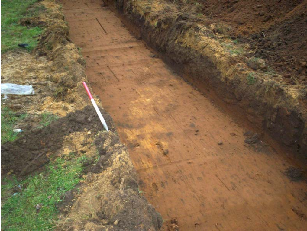
Plate 1. Trench 1, drain cut
