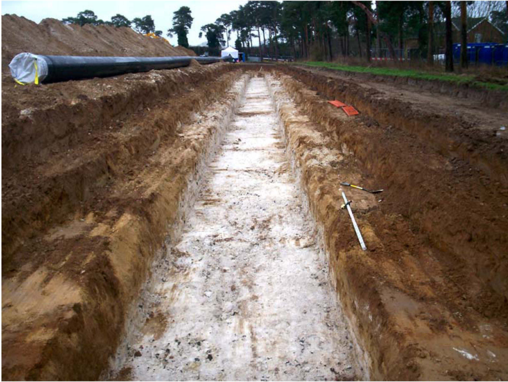
Plate 2. The contact main trench during excavation, facing east
