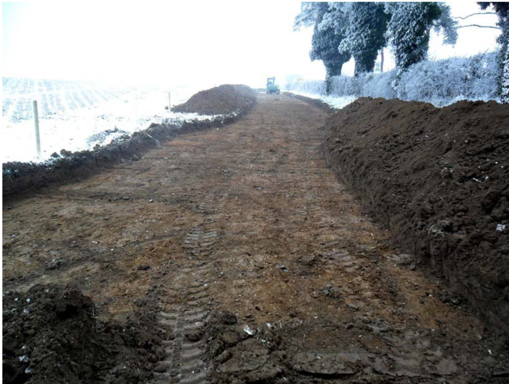
Plate 1. The haul road, facing north
