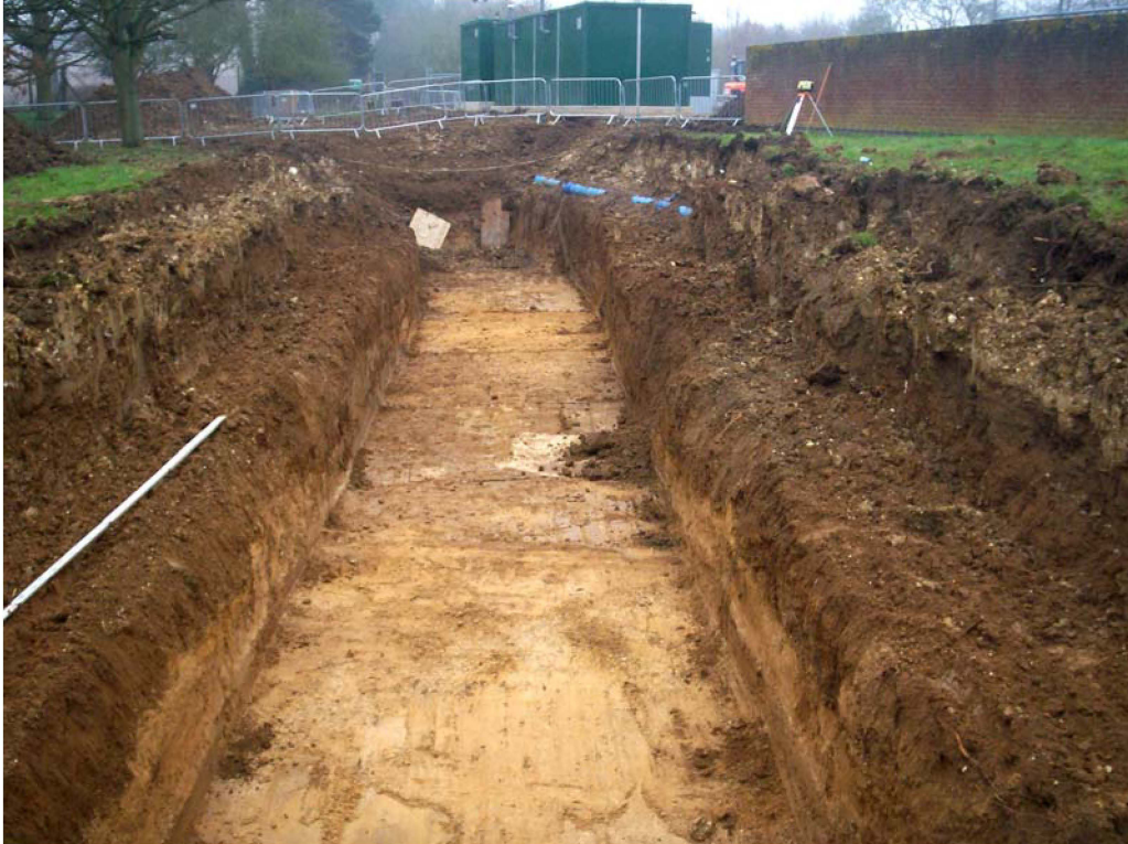
Plate 3. The trench for the linkage pipes, facing south
