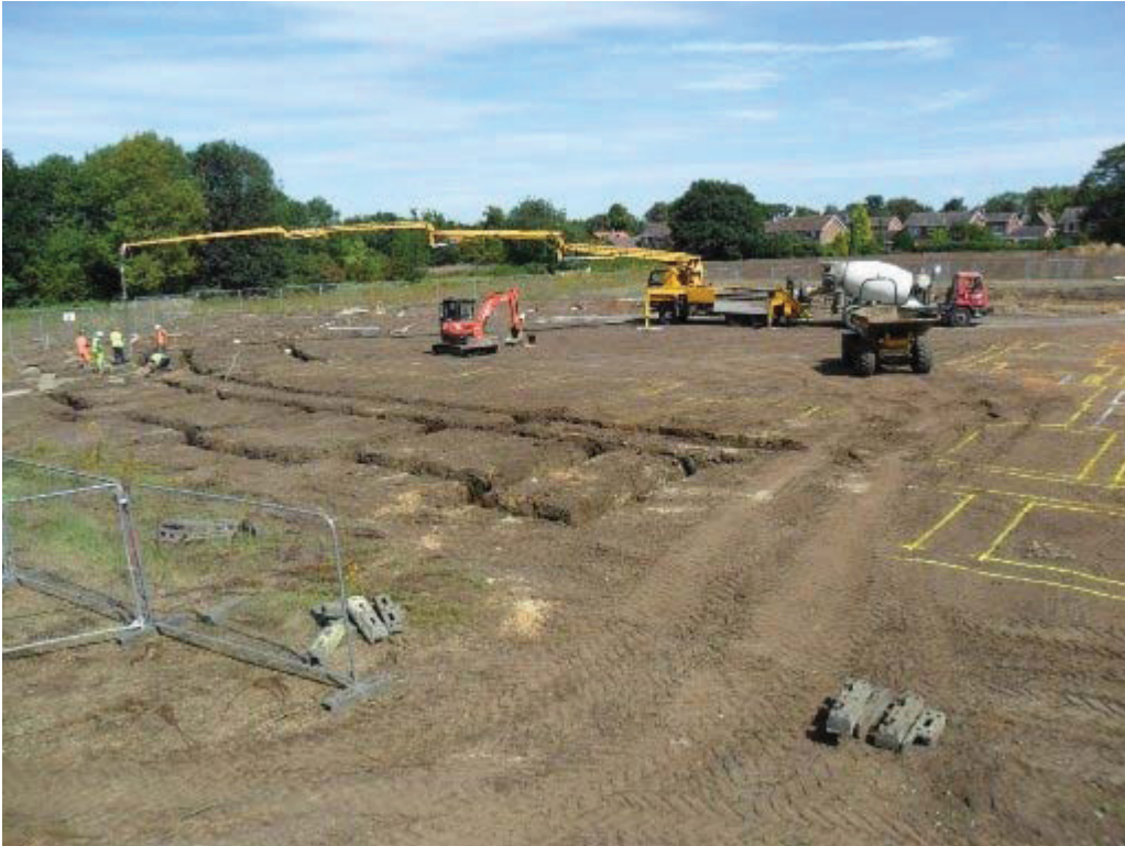
Plate 2. Excavation of footings
