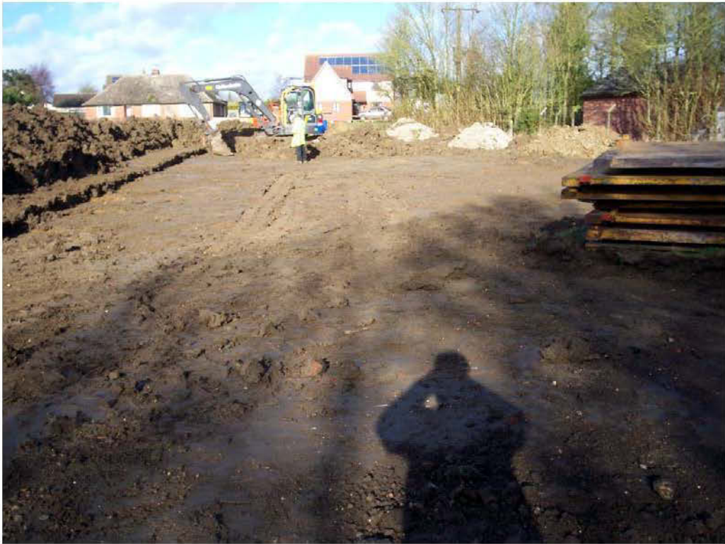
Plate 1. The stripped pumping station area facing north
