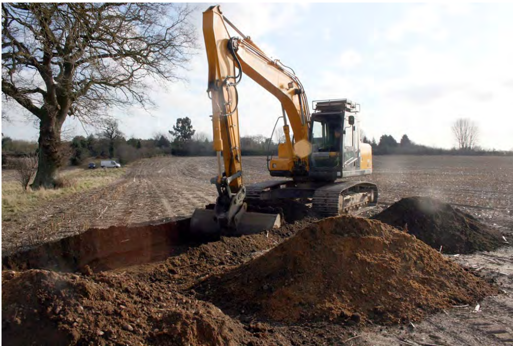
Plate 1. Machining on site, looking east
