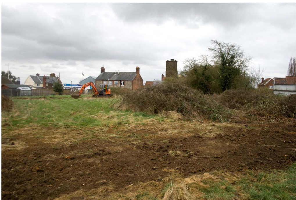
Plate 10. Looking at eastern portion of site during backfilling
