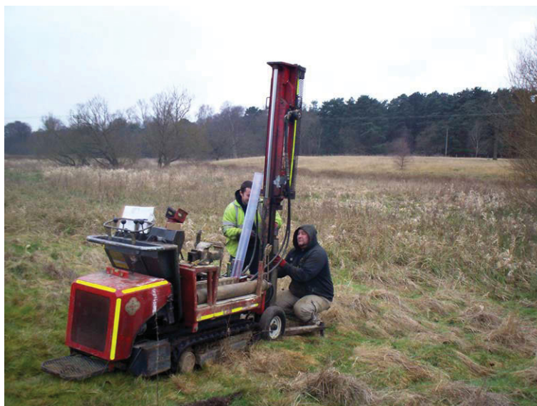
Plate 167. Window sampling rig
